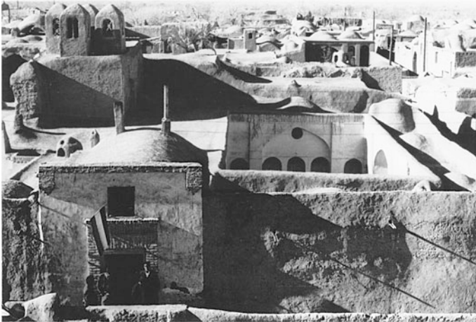
Fig. 6.37 Zaware . Compact structure of the town with low air vent and light inlet
