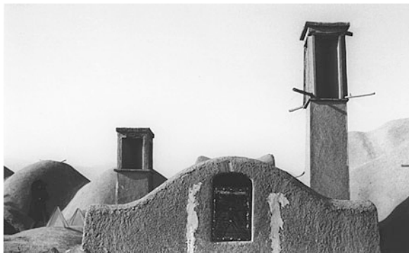
Fig. 6.34 Kashan. Simple four-directional wind catchers
