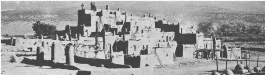
Fig. 7.12 New Mexico. “Structures such as the pueblo of San Juan were constructed of massive adobe roofs and walls, which have good insulative value and the capacity to delay heat impacts for long hours, thus reducing the daily heat peaks. They also used very small windows. By packing buildings together, the amount of exposed surface was reduced. Pueblo structures of this type usually extend on east-west axis, thereby reducing morning and afternoon heat impacts on the two end walls in summer and receiving a maximum amount of south sun in the winter months when its heat is welcome” from Olgyay
