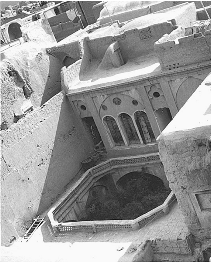
Fig. 6.11 Kashan. Courtyard at two levels, deep shaded structure, hot summer afternoon sun
