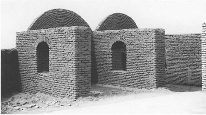
Fig. 6.17 First step in building a simple vaulted roof
