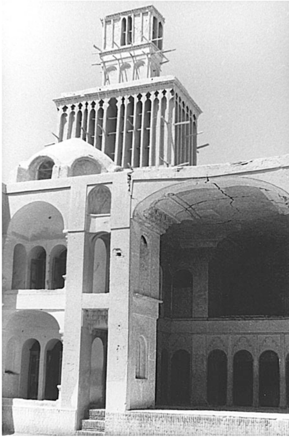
Fig. 6.32 Abarquh. Two-story wind catcher belonging to an aristocratic house
