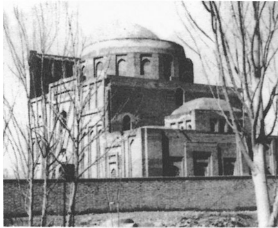
Fig. 6.22 Tus. Harunieh tomb. The external dome is collapsed
