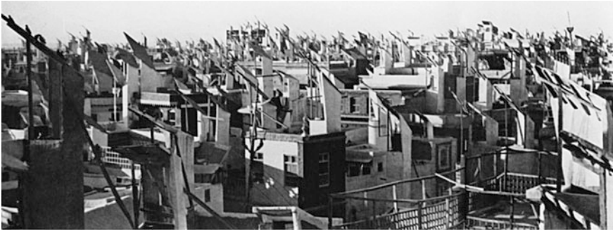
Fig. 7.11 Pakistan. “The air conditioners of Hyderabad Sind. These unusual roofscapes are a prominent feature of the lower Sind district in West Pakistan. From April to June, temperatures range above 120 °F, lowered by an afternoon breeze to a pleasant 95°. To channel the wind into every building, “bad-gir,” wind scoops, are installed on the roofs, one to each room. Since the wind always blows from the same direction, the position of the wind scoops is permanently fixed. In multistoried houses they reach all the way down, ...” from Rudofsky
