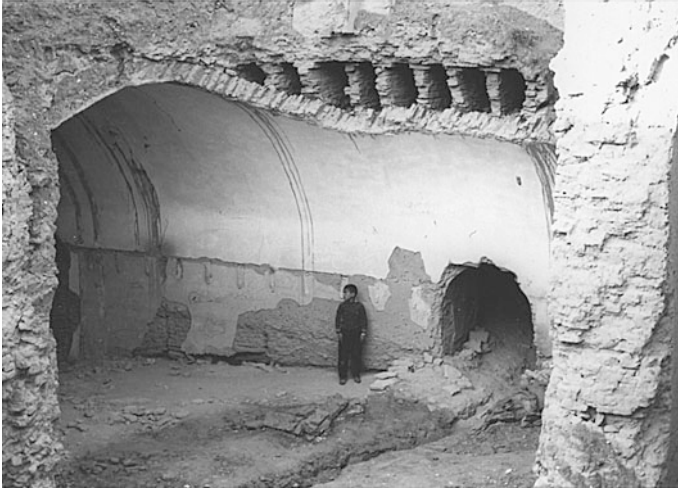
Fig. 6.20 Tabas. The barrel vault of a room with flat roof (partly ruined). The thickness between ceiling and roof is hollow in response to structural problems and thermal insulation
