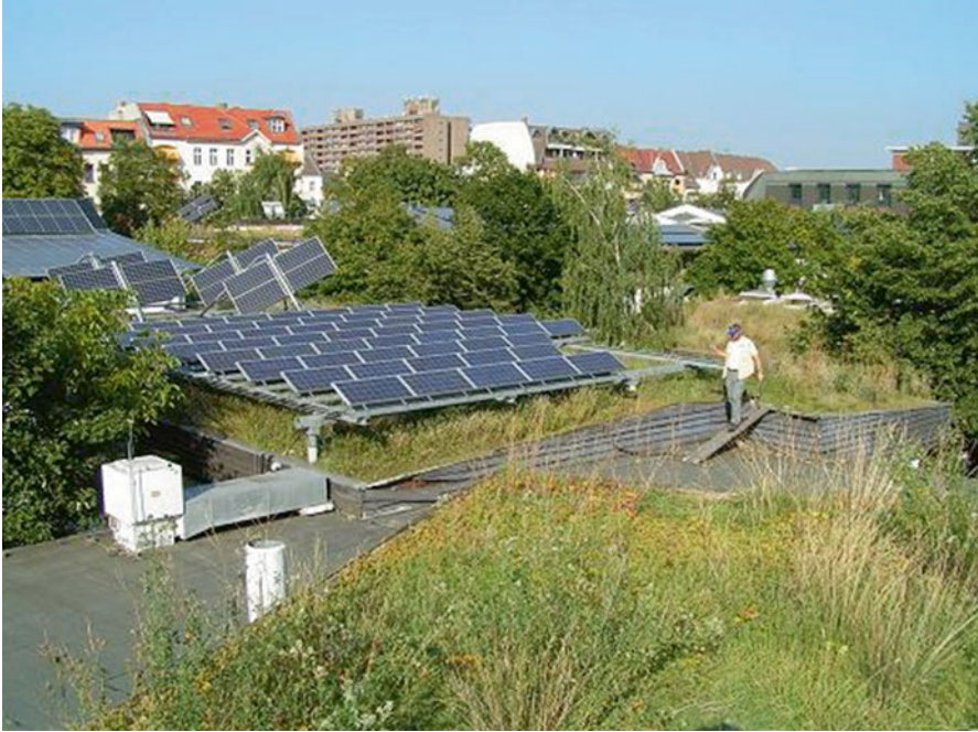
Fig. 19.7 Green roof combined with photovoltaic panels at UFA-Fabrik Berlin-Tempelhof (Photo author)
