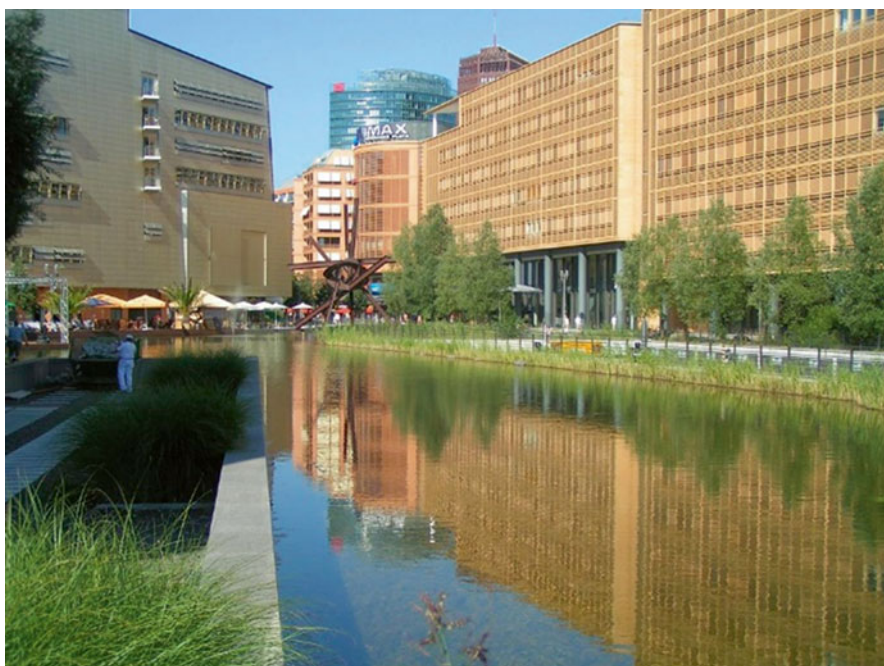
Fig. 19.10 Rainwater retention by an artificial urban lake at Potsdamer Platz, Berlin (Photo author)
