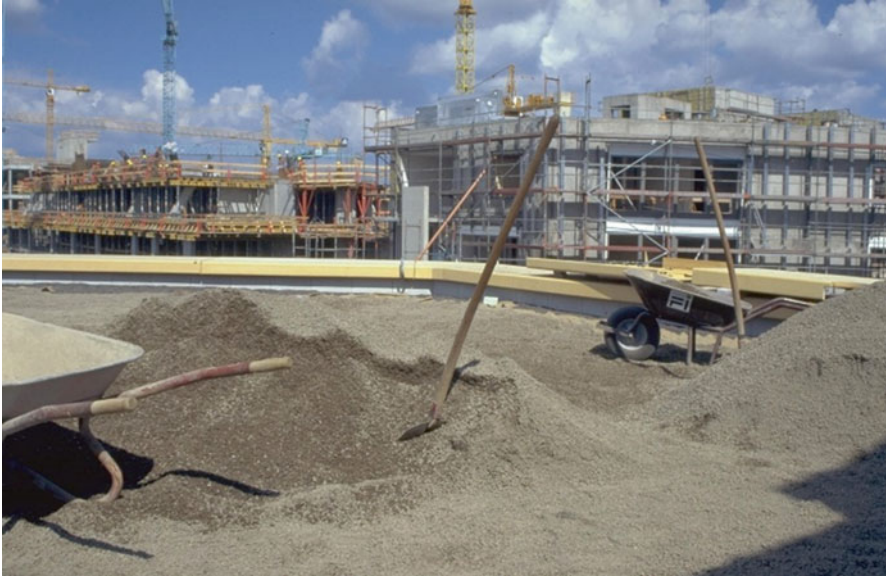
Fig. 19.11 Green roofs at Potsdamer Platz during construction in 1998 (Photo author)
