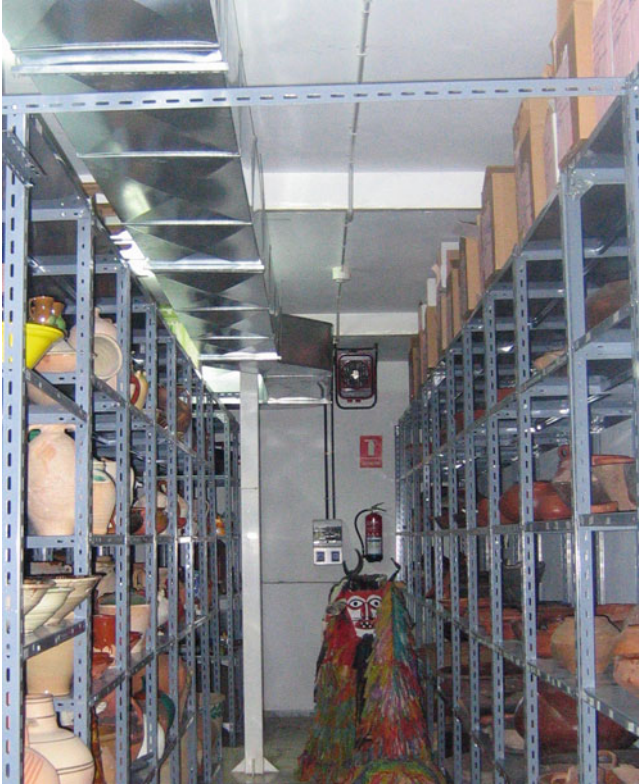
Fig. 9.12 The museum storage in Valle Guerra, Tenerife showing a convective heater on the wall at the far end
