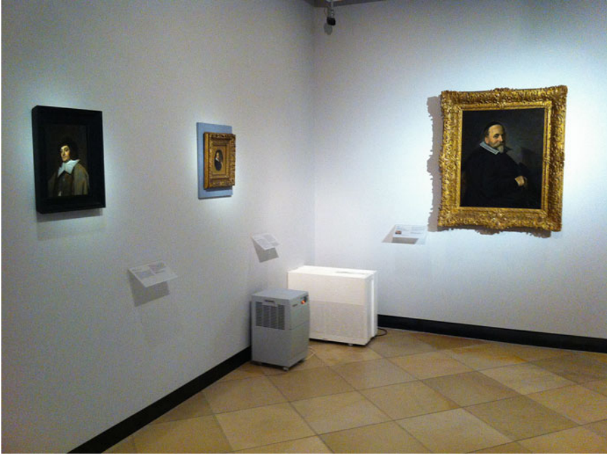
Fig. 9.11 The Frans Hals Museum in Haarlem uses several mobile humidifiers to increase the indoor relative humidity during winter and dehumidifiers to reduce it in summer
