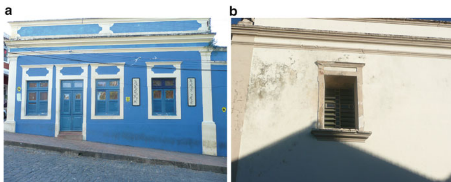
Fig. 7.19 Two buildings in Olinda, Brazil with different types of sun barriers: (a) a dwelling with closed windows (shutters) and doors during daytime and (b) a church window where the glazing system has additional shutters placed to the inside of the building and thus decreasing the sunlit area
