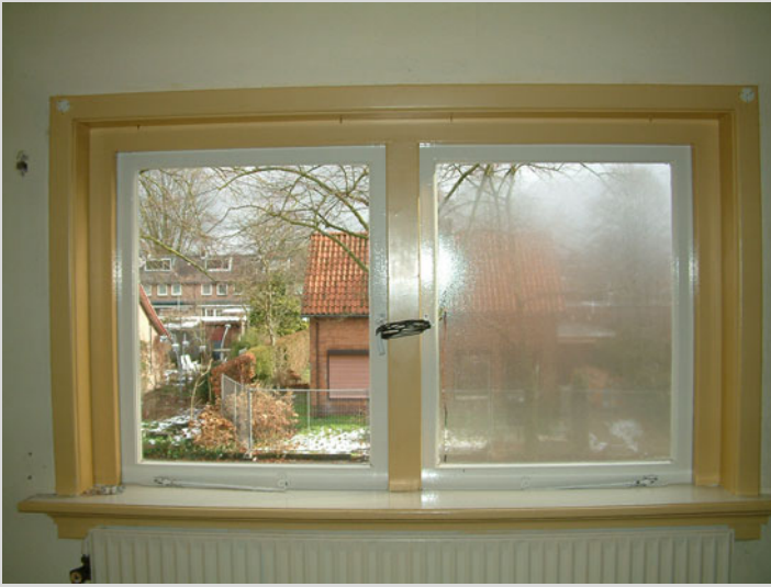
Fig. 7.22 Two window panes in a wooden window frame. The left window is a single clear pane. The right window pane is made of single clear glass coated with a low emissive metal oxide coating on the inside (Photo: H. Schuit 2013)
