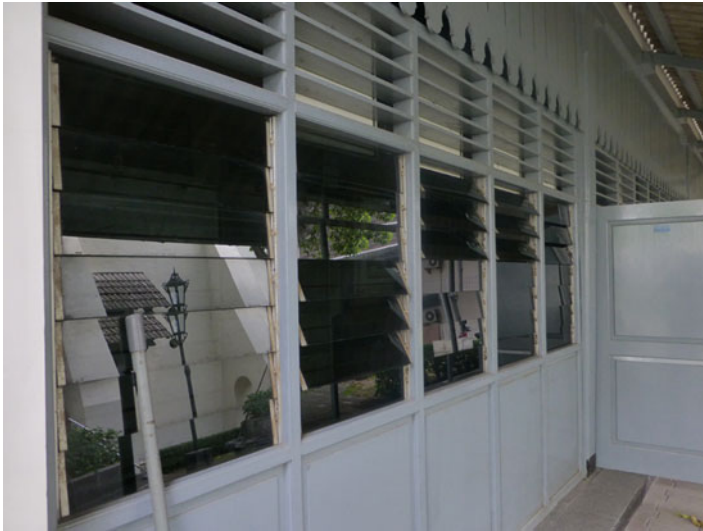
Fig. 7.26 Sometimes ventilation is an easy, cheap and sustainable way to cool and dry the indoor air in tropical regions
