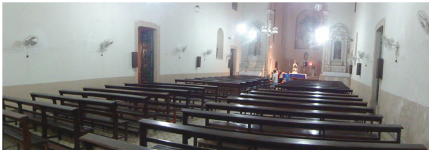
Fig. 6.7 In hot climates options to increase thermal comfort are limited: increasing the air velocity is quite traditional. In this church in Olinda, Brazil, fans are placed on the walls to provide some comfort to the congregation during mass
