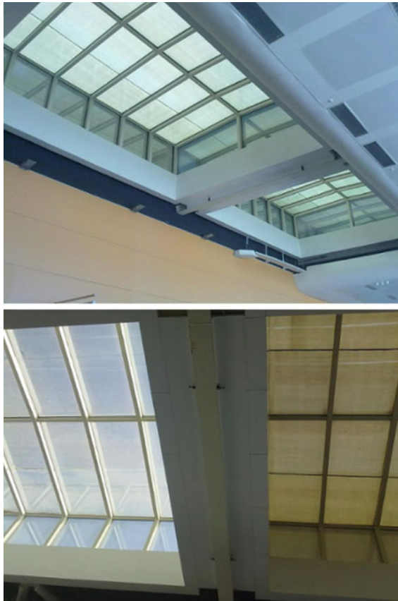
Fig. 7.2 Decorative solar reflective material application on light holes of the terminal
