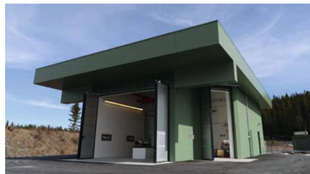
Figure 10 The new test cell for large scale hybrid rocket motor firings (500kN)
