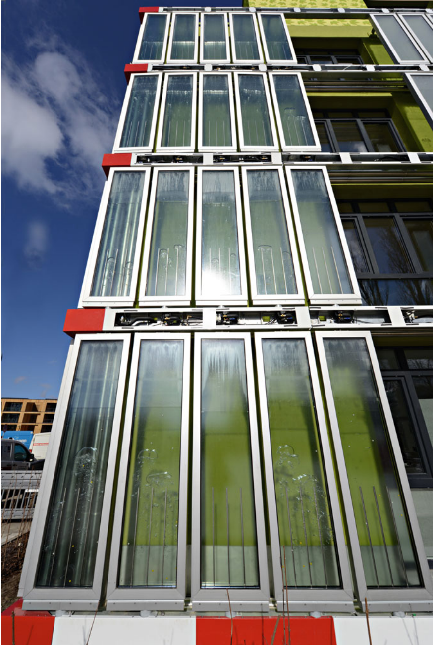
Fig. 31.15 Photograph Colt International. Arup, SSC GmbH. BIQ house that houses microalgae in façade panels containing water. They feed on sunlight and carbon dioxide to produce biomass that is collected, dried and burned back in the building to produce energy that offsets carbon emissions
