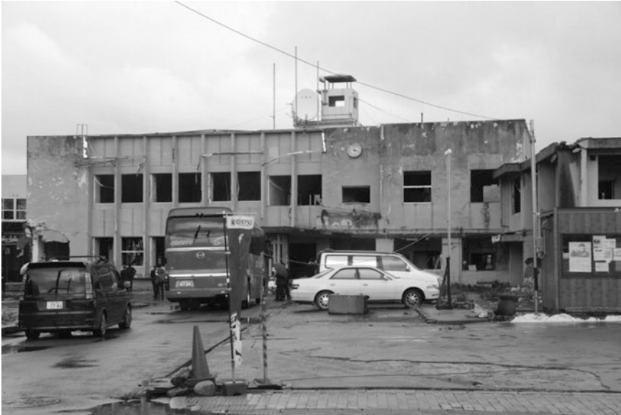
Fig. 4.9 Destroyed town hall building in Otsuchi town
