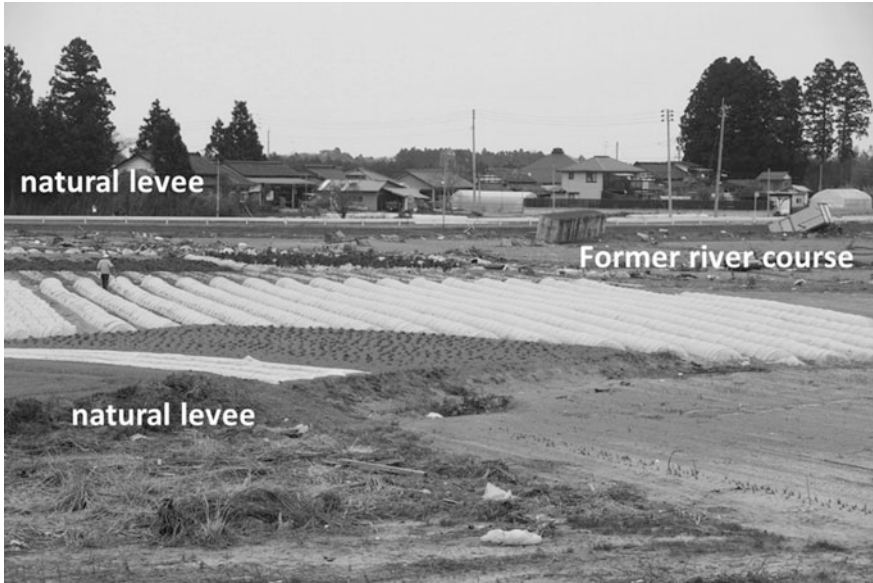
Fig. 4.18 Little damaged old settlement on a natural levee and debris deposited former river course. Many debris including cars and containers were deposited in a former river course
