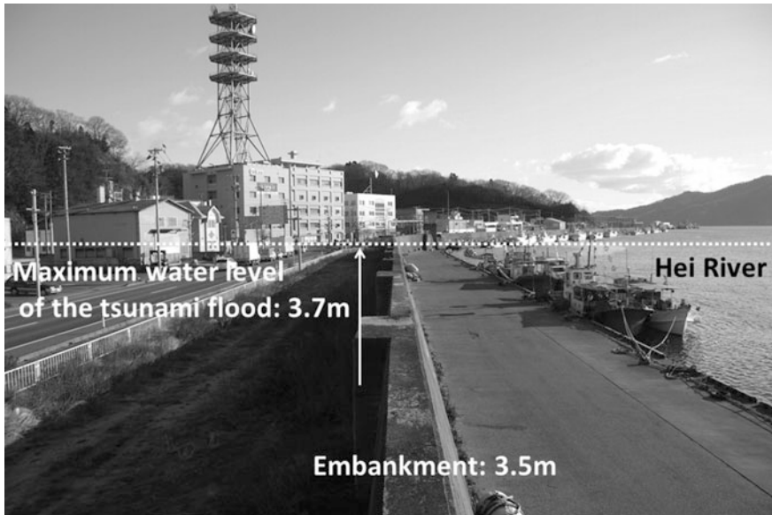
Fig. 4.5 A concrete embankment along the lower Hei River beside the city hall in the Miyako City and the maximum water level of the tsunami flood
