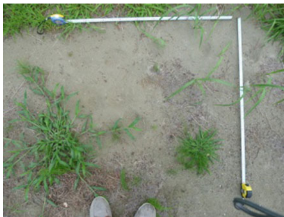
Photo 6.4 Liquefaction points on the boundary line between sand ridge and flood plain at Showa (taken in July 2011)
