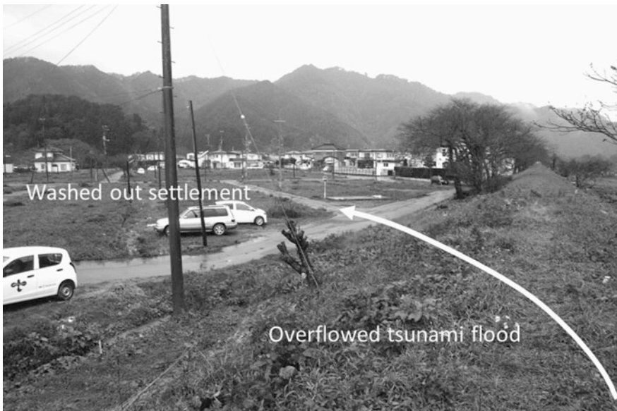
Fig. 4.11 Damaged area caused by overbank tsunami flood flow
