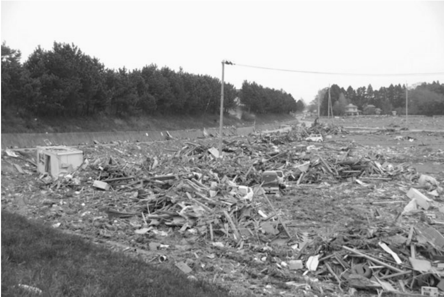
Fig. 4.17 Tsunami dammed up by the elevated motorway. Much debris was deposited along the road
