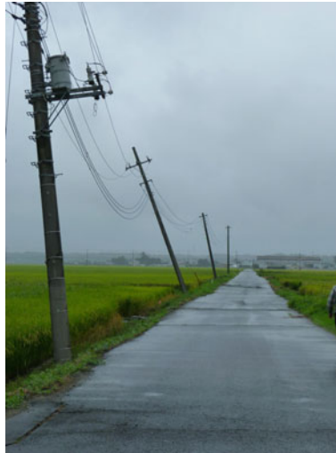
Photo 6.3 Liquefaction of the boundary between natural levee and flood plain at Oogisima (taken in July 2011)
