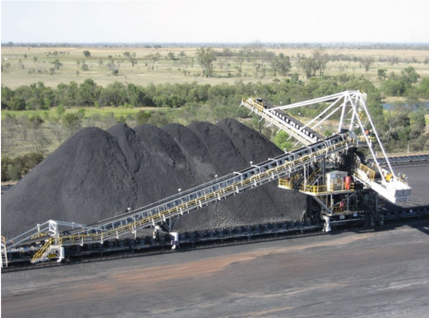
Fig. 1 Conveyor belt system being used in a stacker at a mining site
