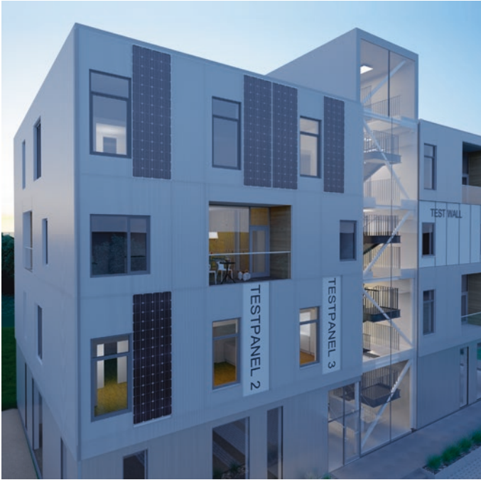
Fig. 10.11 The building includes 12 interchangeable wall/facade test panels that can be replaced through a cassette system, as well as 2 full sections of the façade on the third floor
