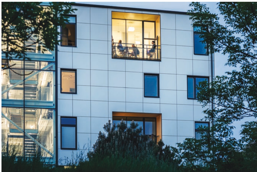
Fig. 10.1 Exterior of HSB Living Lab Version 1.0. The tenants has moved in 1st June 2016
