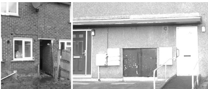
Fig. 11.3 Openings in the thermal envelope. Left to right passageway between terrace houses giving access to back gardens; bin store as internal enclosure between properties
