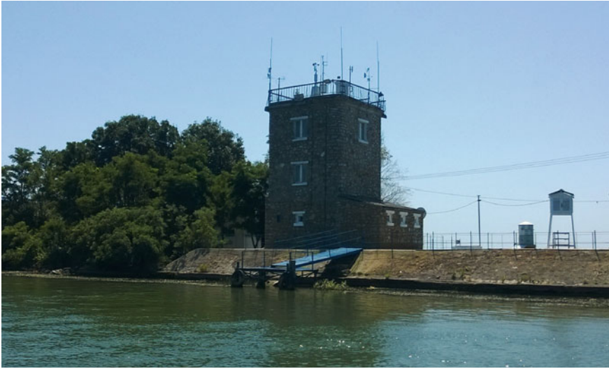
Fig. 34.2 The Sulina meteorological station. The main building sits on top of the Sulina branch jetties. The wind measurement equipment is placed on top of the construction. Photo from the Sulina channel
