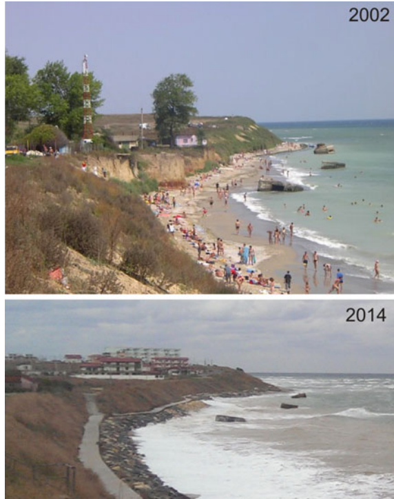
Fig. 24.6 Intense erosion in the northern sector of Costinești ( -2 m/year). Bunkers from the Second World War were installed initially at the cliff base. New restoration projects were made in the Past years involving sea walls and rock armor in the cliff base, but the anthropogenic pressure increased on the tableland
