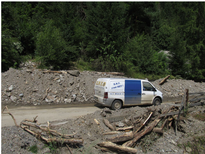
Fig. 14.8 County Road covered by debris. The image shows the state after authorities' intervention which cut a breach in the debris deposit (photo taken in July 2014 by V. Ilinca)
