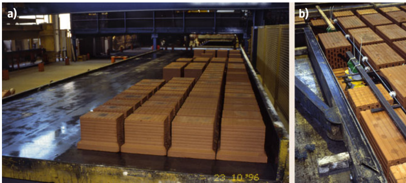
Fig. 57.8 (a) Automated horizontal brickwork layering robot station; (b) insertion of reinforcement and house infrastructure
