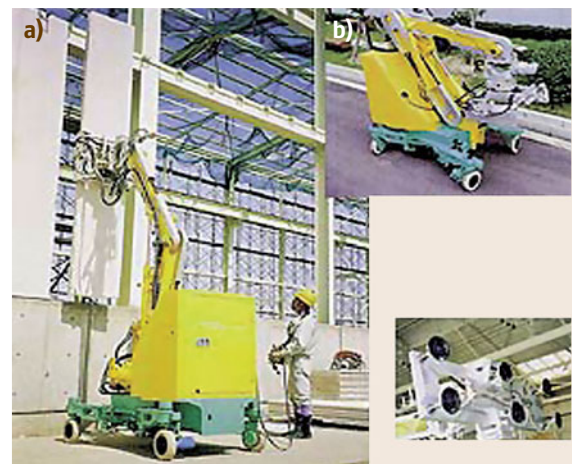
Fig. 57.22 Concrete panel installation robot (courtesy of Fujita Research)
