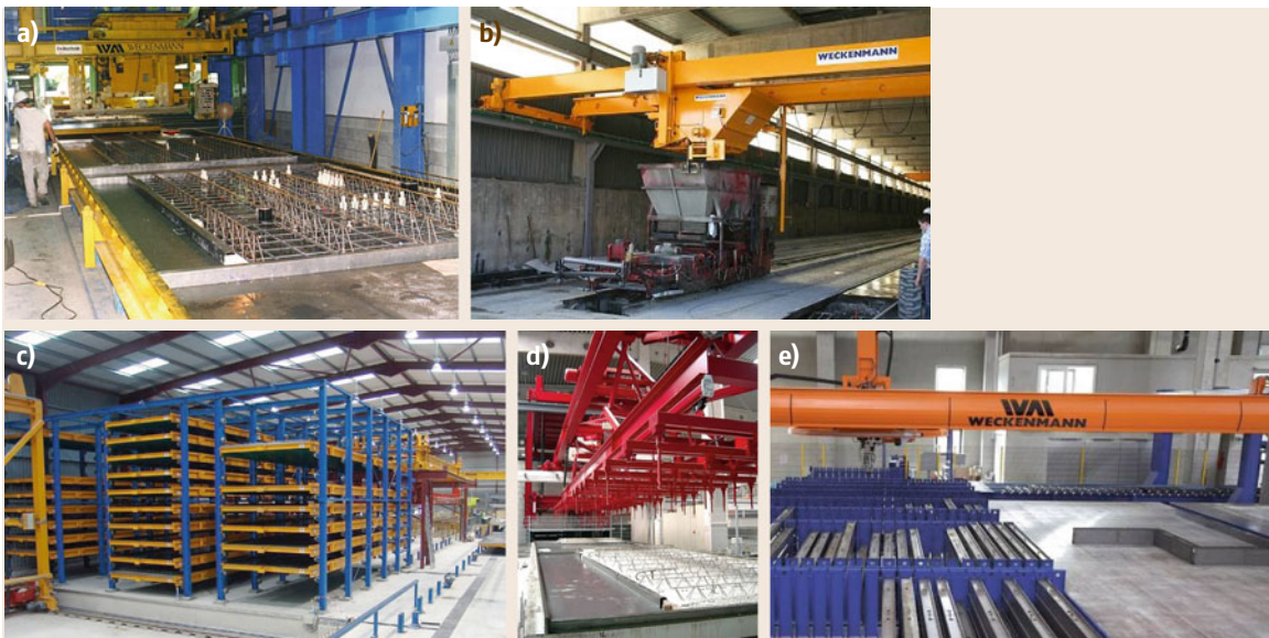
Fig. 57.2 (a) Pallet in concreting station; (b) bridge crane; (c) pallets molding systems; (d) demolding-depalletizing device; (e) cleaning, measuring and oiling (after [57.42])
