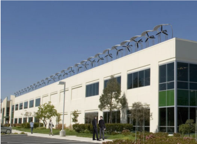
Fig. 9.8 Horizontal axis wind turbine installed on a building in urban settings with gear box assembly and generator fixed on the rotor (Atmospheric Water Systems, Inc. 2010)
