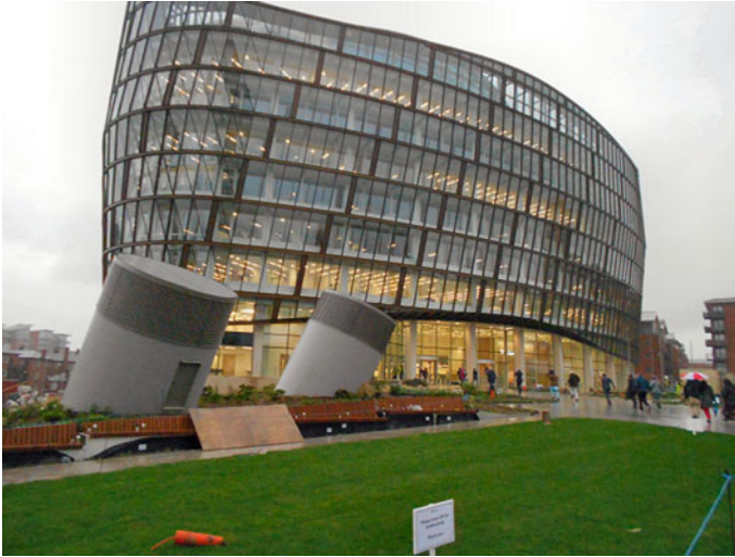
Fig. 8.8 Earth cooling tubes, one angel square, Manchester, UK (Dixon 2012)
