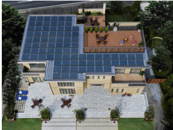
Fig. 12.6 Modular housing rooftop PV Arrays (Sekisui Chemical Co. Ltd.)
