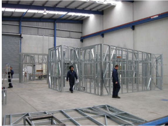
Fig. 3.1 Precut light gauge steel components assembled as house framework (Kiwi Prefab 2012)
