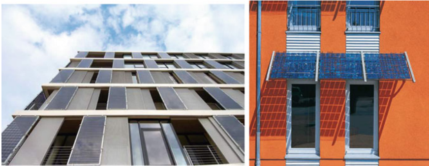
Fig. 9.32 (Left) PV panels as window shutters, (Colt international 2011); (right) Solar awnings, (Solar Awning inbalance-energy.co.uk)
