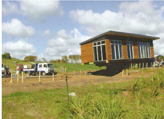
Fig. 3.5 A completed building arrives at site on the back of a truck (Kiwi Prefab 2012)
