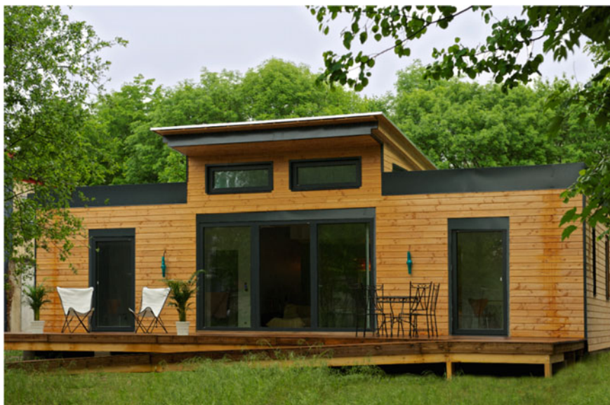
Fig. 10.8 Vermont House by ECOxIA: positive energy Vermont House in Yverres, France
