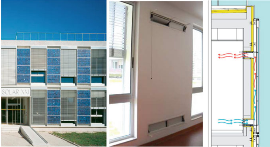
Fig. 9.35 Solar XXI BIPVT system: (Left) façade, (middle) operable vents behind BIPVT, and (right) Schematic diagram showing flow direction of air (Aelenei and Gonçalves 2014)
