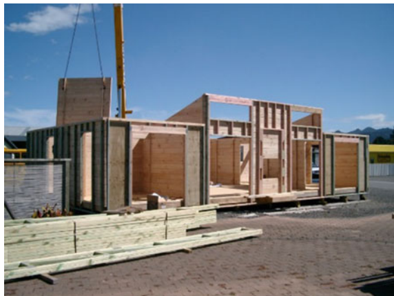
Fig. 3.2 Timber panels assembled as house structure (Kiwi Prefab 2012)
