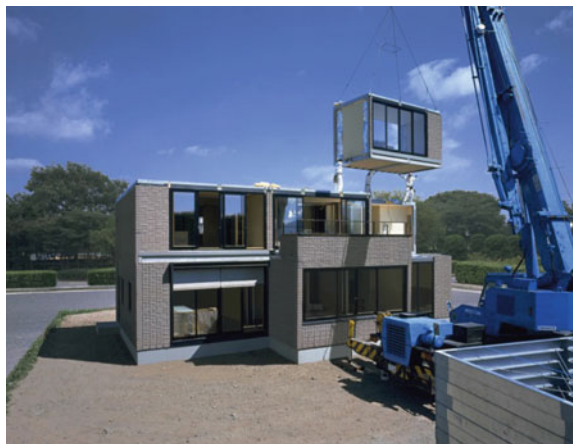
Fig. 12.3 Modular housing on-site assembly (Misawa Homes Co. Ltd.)
