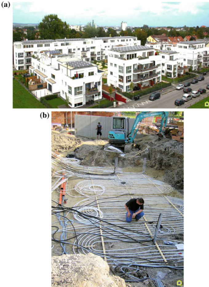
Fig. 9.13 a View of Landhut Ludmilla residential site. b Laying the measurement technology for the ground collectors (Landhut 2015)
