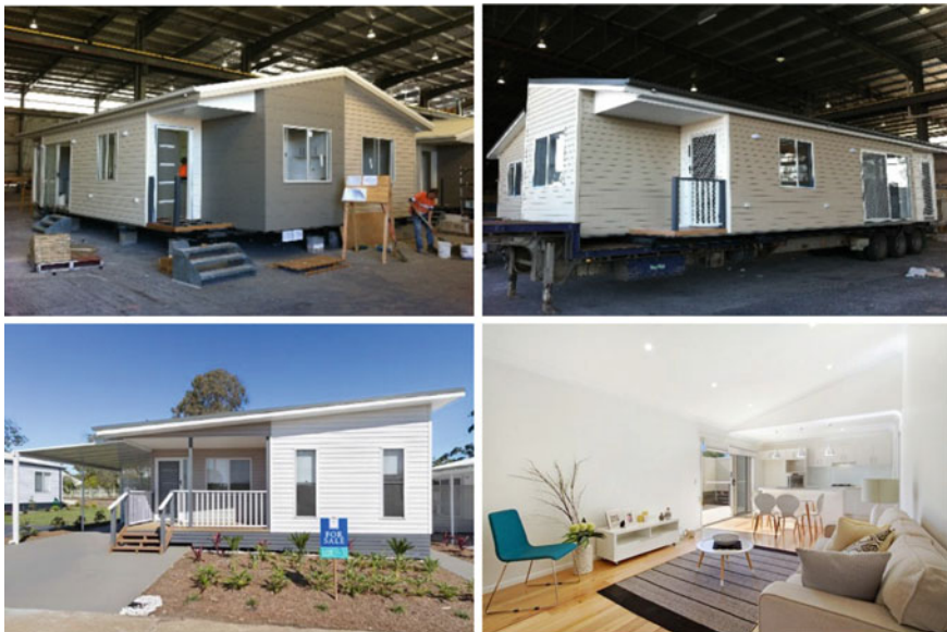
Fig. 3.9 A single storey 120 m 2 , two bedroom house in factory, transport ready, and as delivered on site. The entire construction process from initial order to completion in the factory has been six weeks/30 working days (Fleetwood AU)
