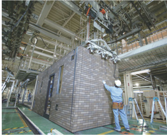
Fig. 12.2 Modular housing unit in-factory assembly (Sekisui Chemical Co. Ltd.)
