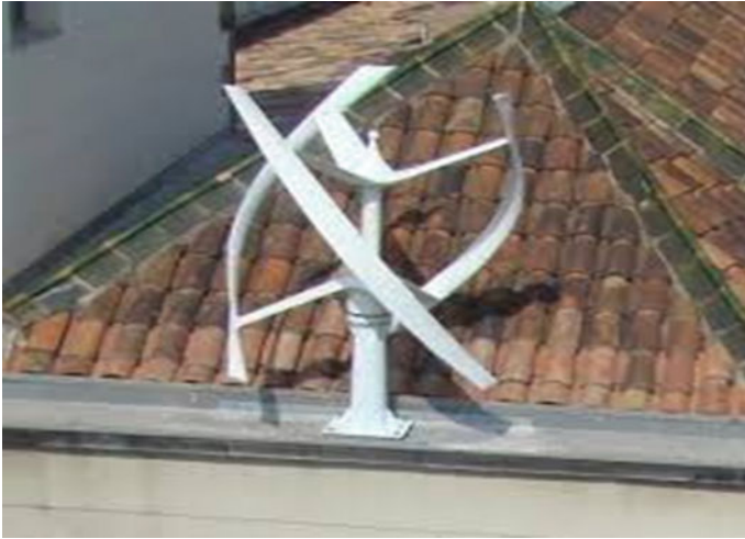
Fig. 9.9 Vertical axis wind turbine installed on the roof (Keough et al. 2014)
