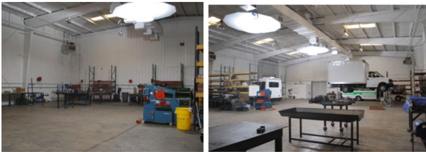
Fig. 9.21 Warehouse daylighting with Sundolier systems Loveland, Colorado (Sundolier 2015)
