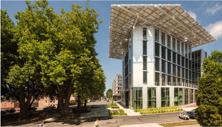
Fig. 11.7 Bullitt Centre, Seattle: example of net zero energy building with integrated PV roof (Bullitt Centre 2015)
