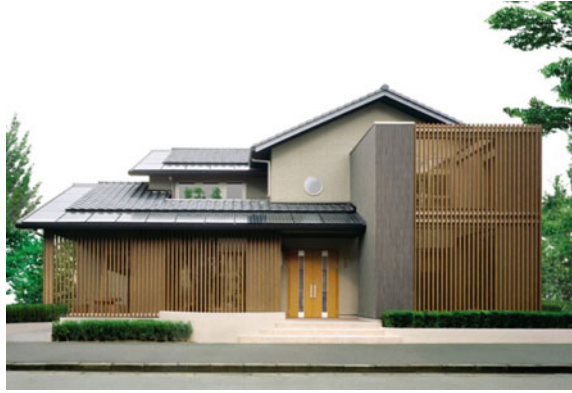
Fig. 12.9 Building integrated PV (Sanyo Homes Corp.)
