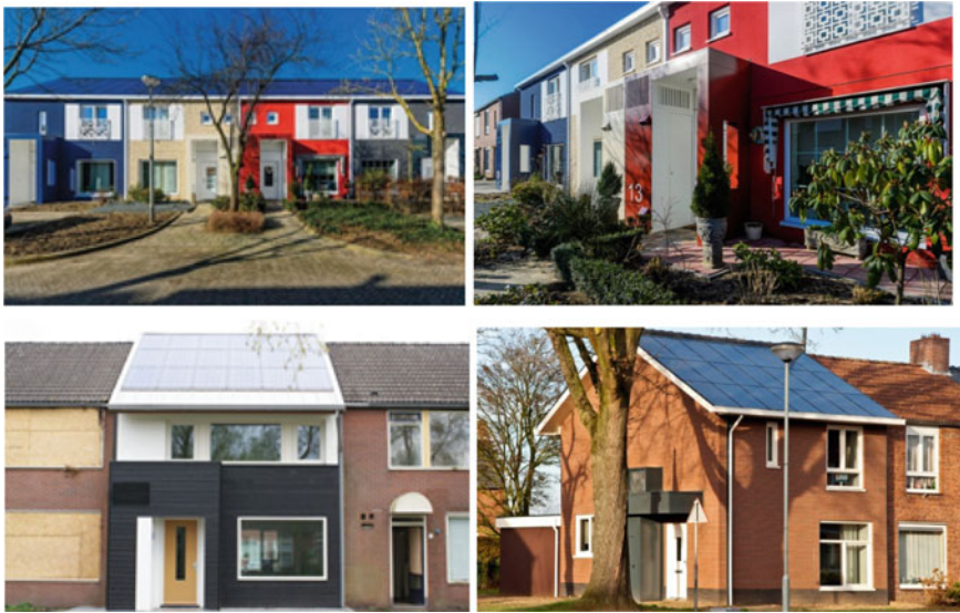
Fig. 10.19 Examples of mass housing retrofitting in the Netherlands (Energiesprong 2015a, b)
