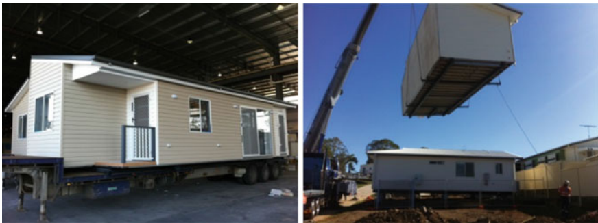
Fig. 3.16 Units are loaded on a trailer. Unit sizes vary and are governed by local government road regulations. A unit size of 4.2 \times 14.4 m is an economical dimension which can reduce material waste and transportation costs. Site location and surrounding environment, road conditions from factory to site, and local road regulations should be checked prior to design of module sizes
