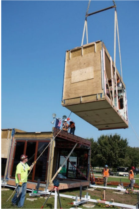
Fig. 3.3 Modular volumes being set into position on site (Kiwi Prefab 2012)
