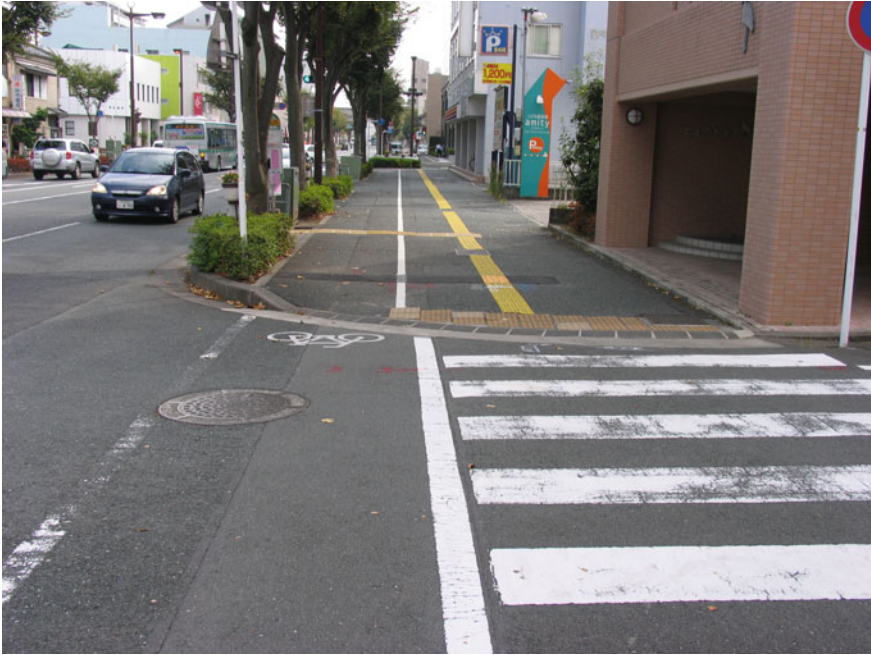
Fig. 6.2 Tactile pavement and ramps for easy access and mobility
