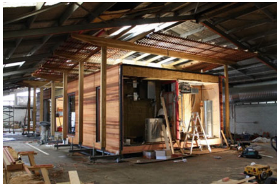
Fig. 3.7 Off-site undercover construction (Kiwi Prefab 2012)
