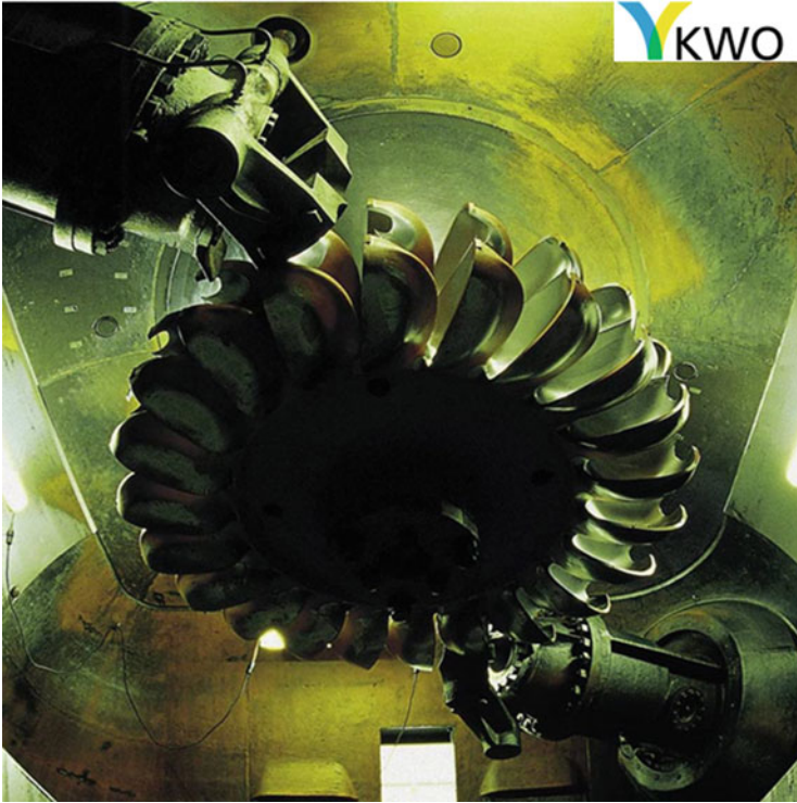
Fig. 1.1 Two-injector Pelton turbine installed at the Oberhasli Hydroelectric Power Company (KWO). Pressure head H = 670\text{m} , flow rate \dot{Q} = 8.25\text{ m}^3/\text{s} , rotational speed n = 428.6\text{rpm} , power output P = 48.6\text{MW}
