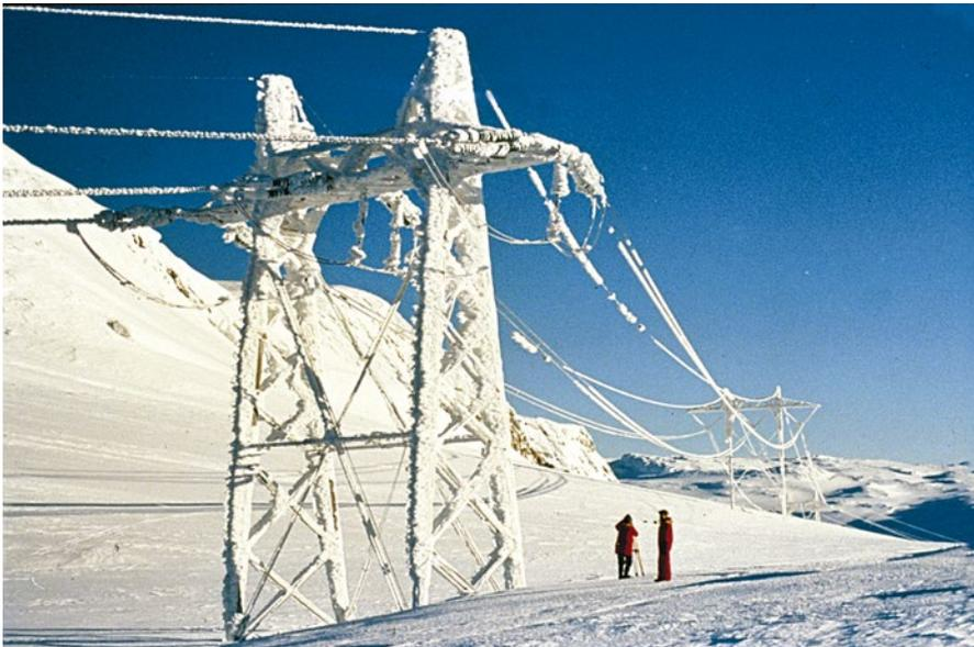
**Figure 7.13** Rime icing on a 420 kV line in Norway, 1400 m above sea level (Photo: S.E. Hagen).
