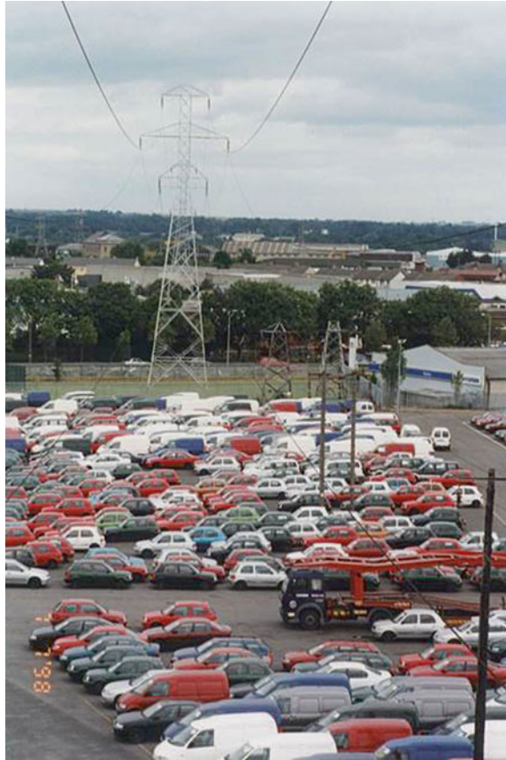
Figure 6.7 A double circuit 110 kV line corridor used as a car park in an industrial area (Ireland).
