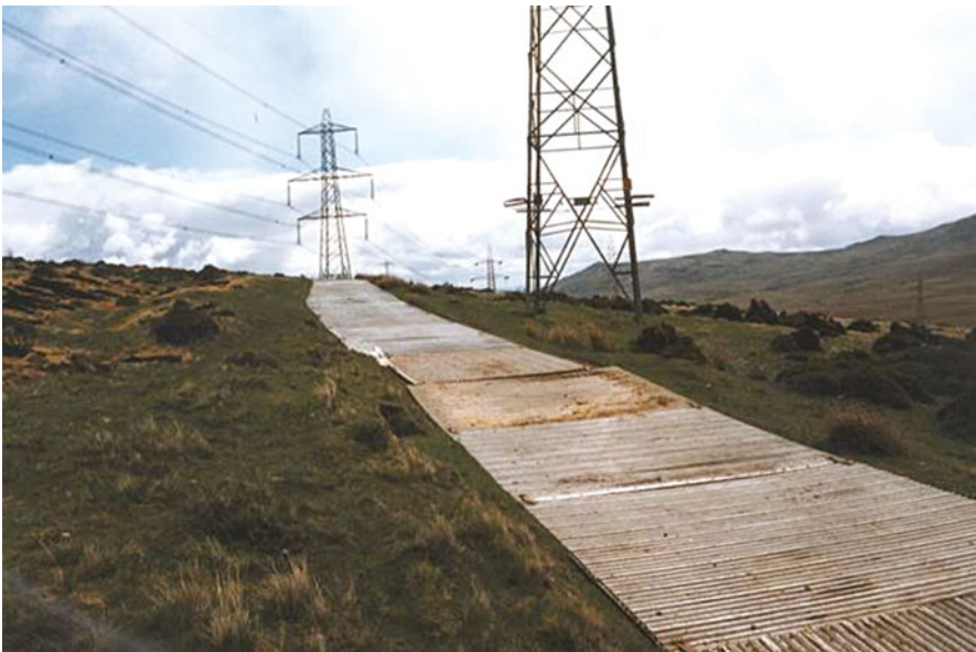
Figure 6.9 Special Temporary Trackway (England).
