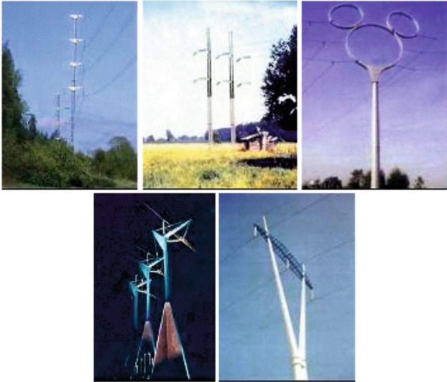
Figure 19.10 New tower design; from left: Finland, France, USA, Finland, Spain (Source: Cigré TB 416).
