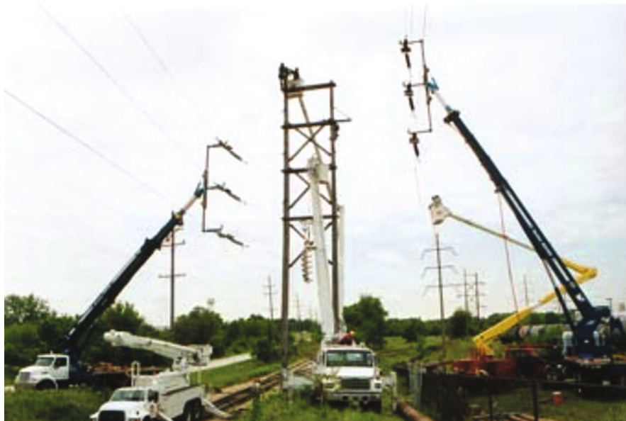
Figure 16.15 Photo of the boom truck and LineMaster™ in action.
