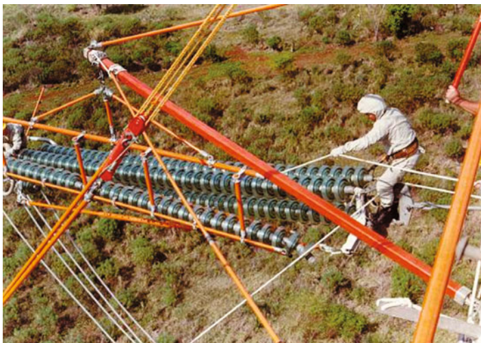
Figure 16.13 Changing 600 kV Insulator String using Bare Hand Method (Brazil).
