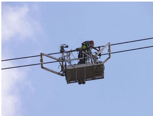
Figure 16.10 Cart used on a horizontal twin bundle.
