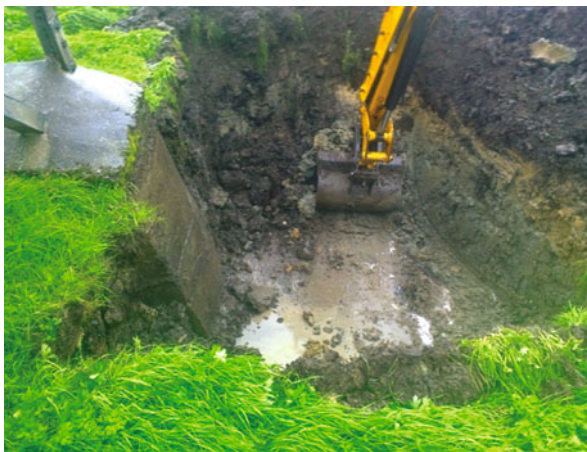
Figure 16.9 Foundation condition below ground.
