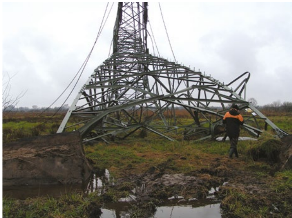
Figure 15.9 Destroyed tension tower of a 220 kV OHL.
