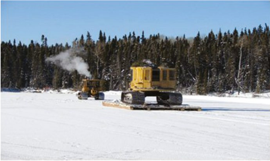
Figure 15.3 Transportation of heavy construction equipment over a frozen lake.
