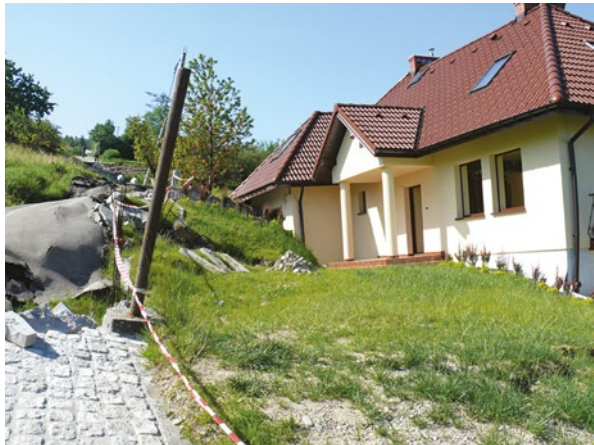
Figure 15.12 Landslide causing destruction of a road, a house and a tower on a 110 kV OHL.
