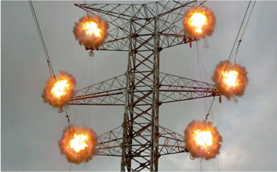
Figure 15.43 Simultaneous installation of multiple implosive type sleeves.
