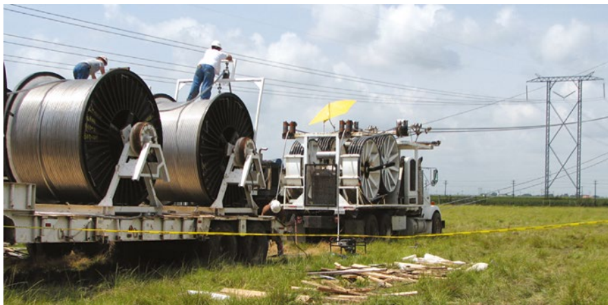
Figure 15.33 Trailer mounted payoffs and a truck mounted bullwheel for tension stringing (Courtesy of Southwire Co.)
