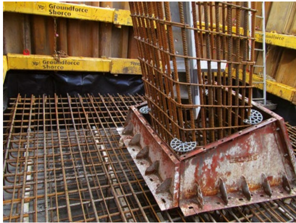
Figure 13.52 Steel formwork.
