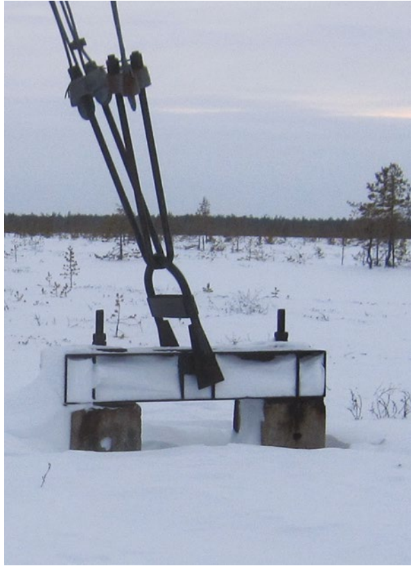
Figure 13.24 Pre-cast concrete pile – Portal guyed tower guy anchor.
