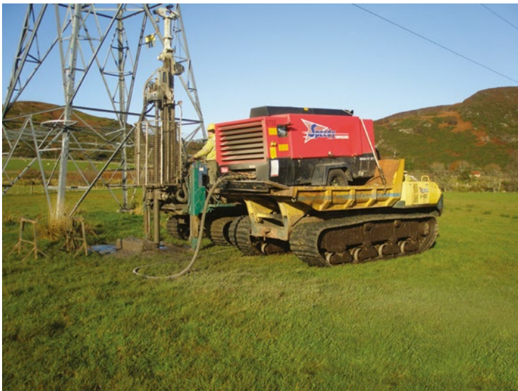
Figure 13.64 Foundation upgrading – Installation of micropiles.
