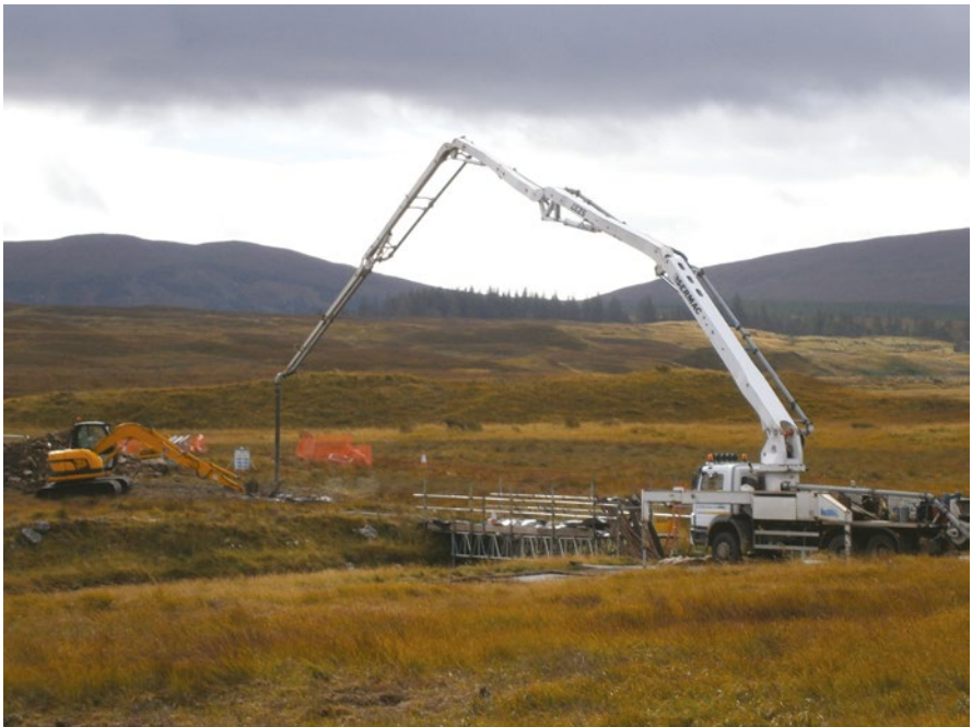
Figure 13.57 Placing of concrete using a concrete pump.
