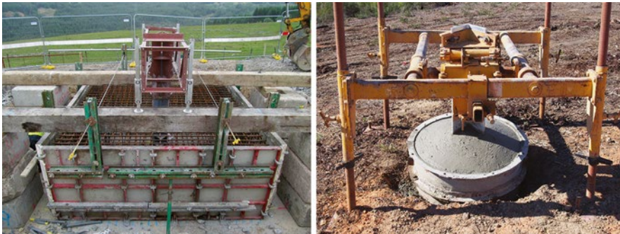
Figure 13.55 Stub setting.
