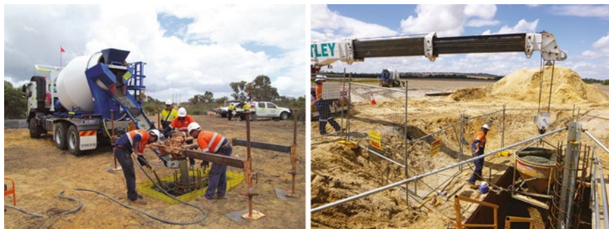
Figure 13.58 Placing of concrete using chute (left) and skip (right).
