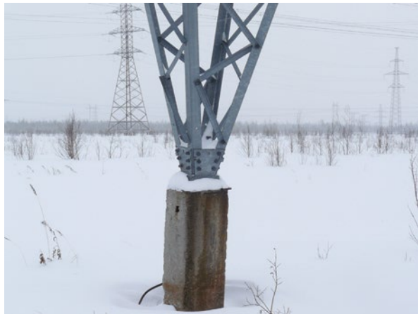
Figure 13.23 Pre-cast concrete pile – Portal guyed tower mast base.
