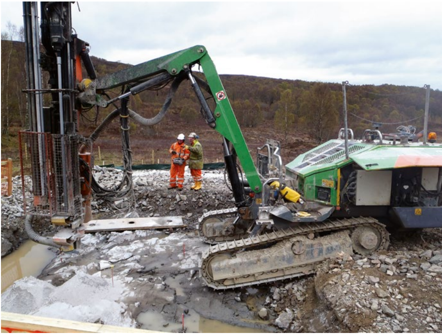
Figure 13.51 Rock anchor installation.
