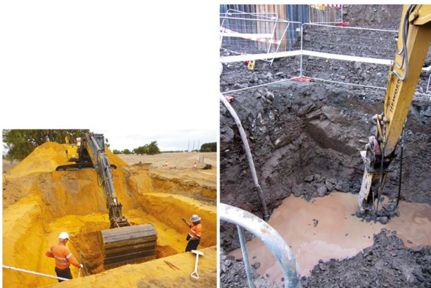
Figure 13.48 Foundation excavation in soil (left) and rock (right).
