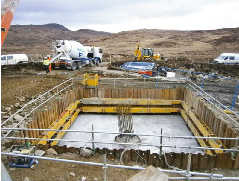
Figure 13.54 Intermediate stage concrete pad cast prior to placing stub and chimney formwork.
