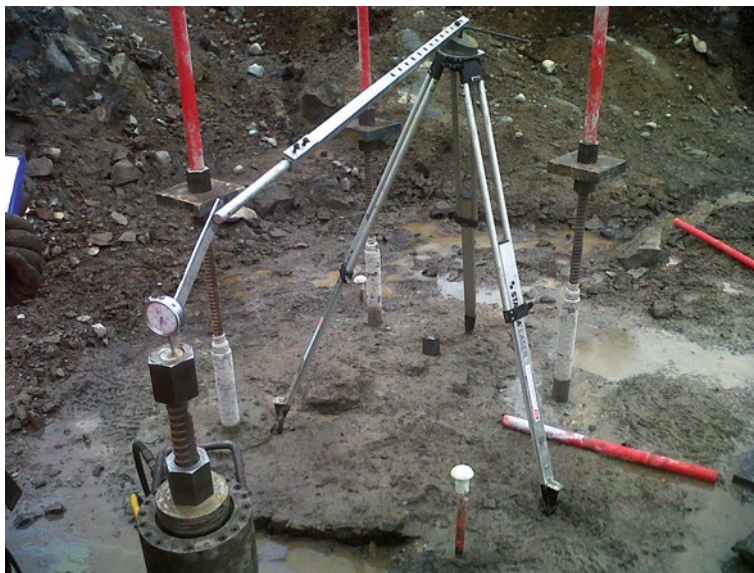
Figure 13.44 Proof testing of individual rock anchors.
