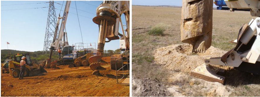
Figure 13.49 Installation of Bored piles.
