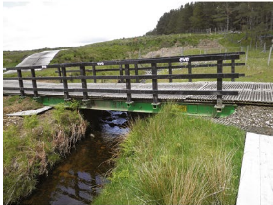
b) Temporary access track using aluminium track way panels and temporary bridging over a stream
