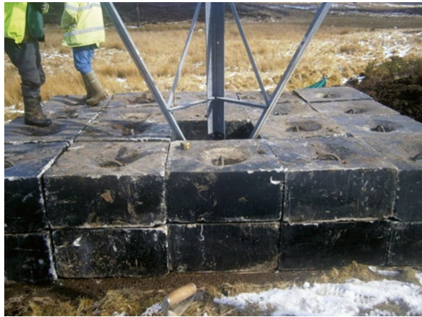
Figure 13.63 Foundation upgrade – Use of precast concrete blocks.
