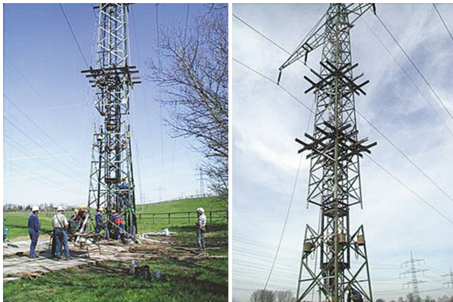
Figure 12.105 Replacement of main members.
