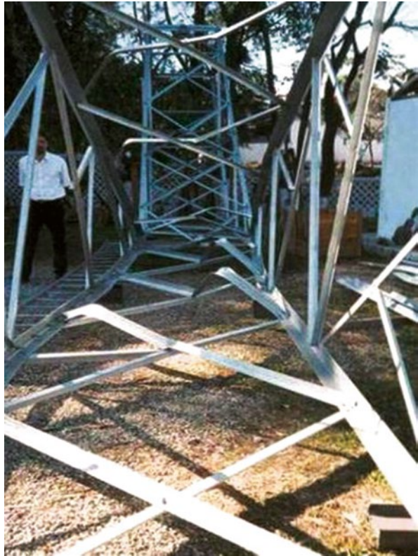
Figure 12.25 Diagonals buckling during test. (See the bracing provided by the tension diagonals)
