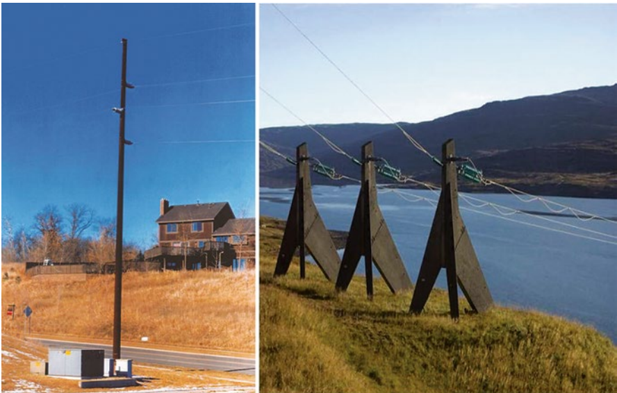
Figure 12.9 Wood OHL Supports.
