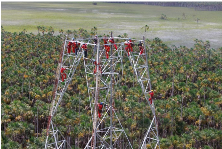
Figure 12.11 Workers on the support during tower erection.
