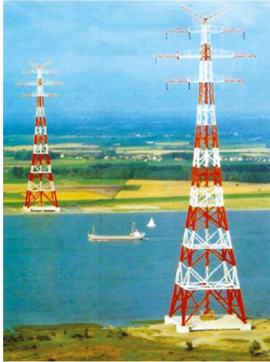
Figure 12.69 4 \times 380 kV - Elbe River Crossing, Germany.
