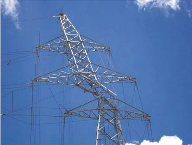
Figure 12.57 Destructive test – 230 kV Double Circuit tower.
