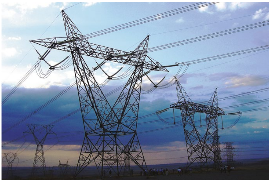
Figure 12.2 500 kV Anchorage Tower.
