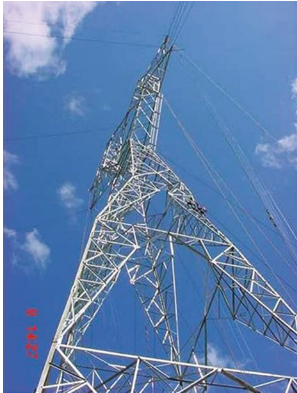
Figure 12.56 Failure at 100% loading step.
