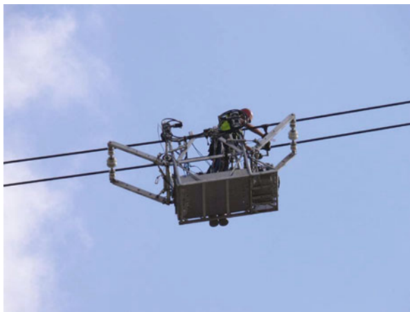
Figure 1.22 Cart used on a horizontal twin bundle.
