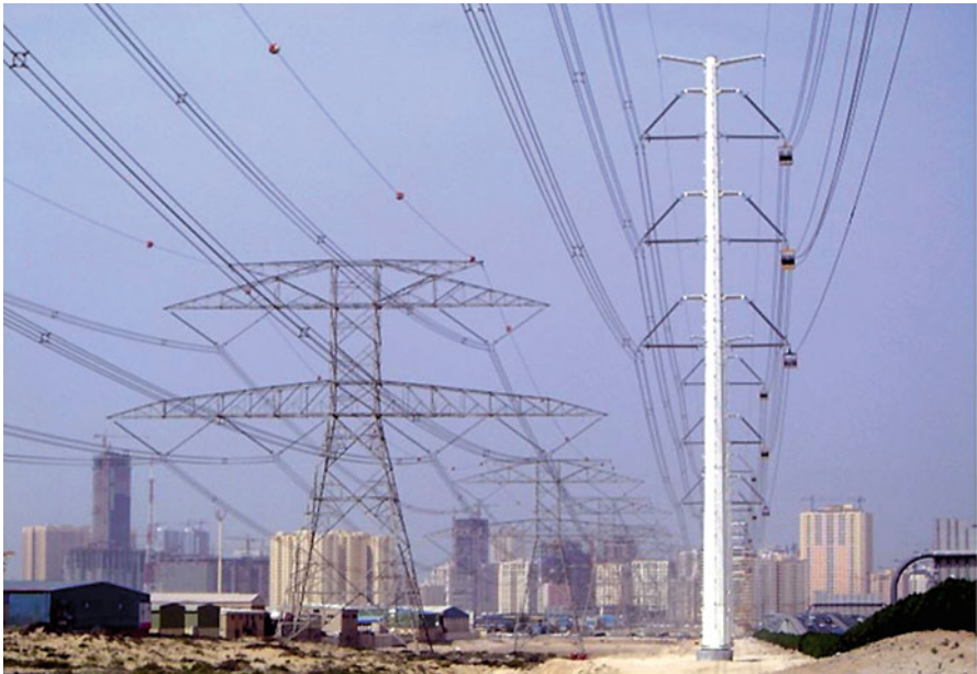
Figure 1.16 Visual comparison of 420 kV conventional and compact lines side by side carrying the same power in Dubai/UAE.
