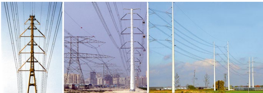
Figure 11.71 Swiss 420 kV horizontal Vee, commissioned in 1998 ( left ), DEWA's 420 kV horizontal Vee, commissioned in 2007 ( middle ) and the Dutch 420 kV horizontal Vee solution of TenneT, commissioned in 2011 ( right ).
