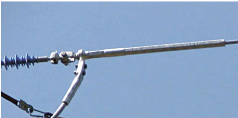
Figure 9.71 Die compression clamp.
