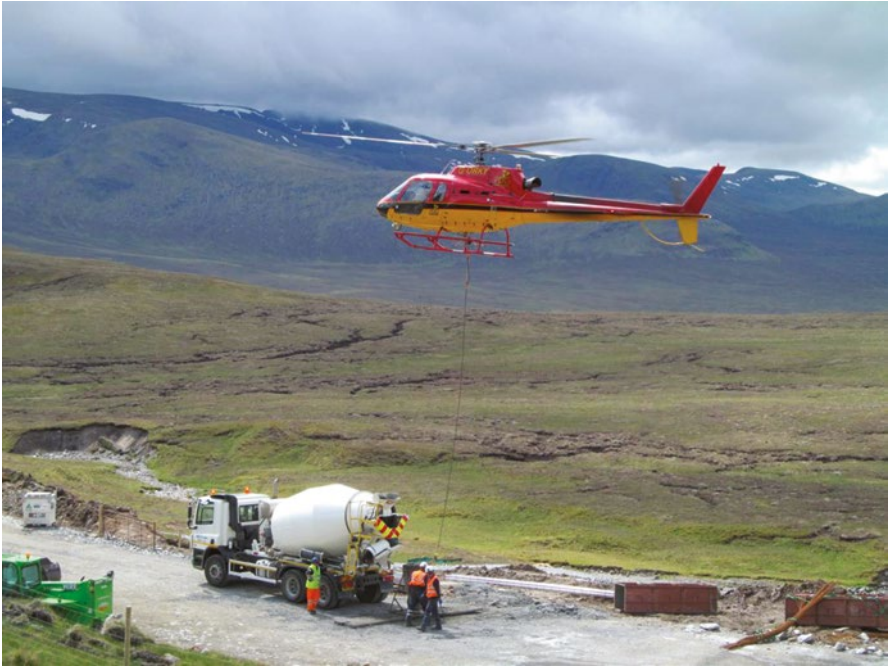
Figure 13.56 Transportation of concrete – helicopter.
