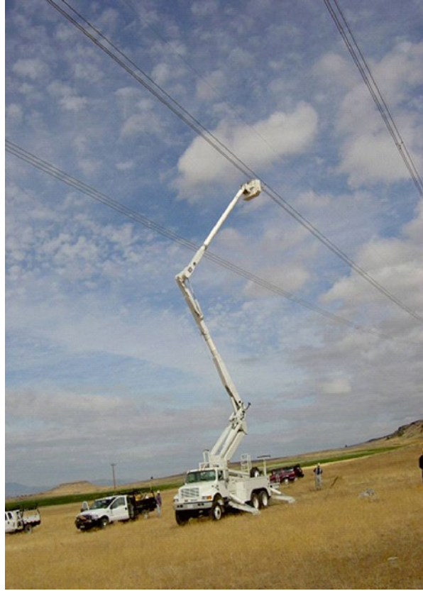
Figure 9.28 Bucket truck used for installation of spacer dampers.
