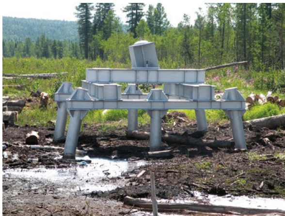
Figure 13.22 Steel screw piles with steel grillage – 500 kV portal guyed tower mast base.
