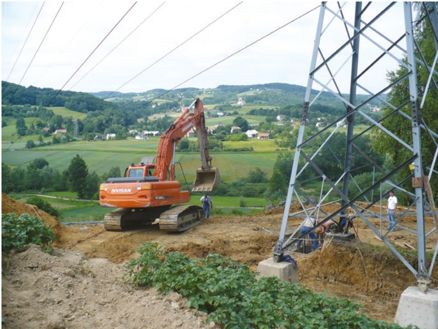
Figure 15.5 Hydraulic excavator during the work of strengthening the foundation of 110 kV OHL.
