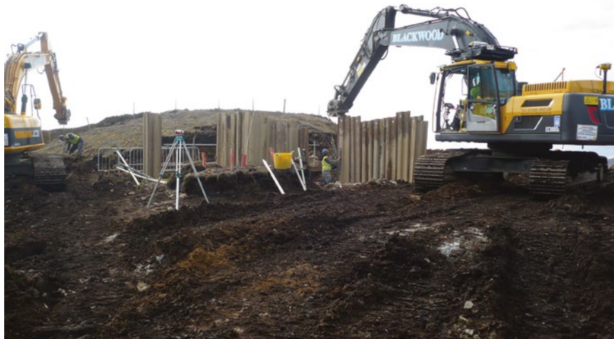
Figure 13.47 Foundation excavation installation of temporary support system (sheet steel piles).
