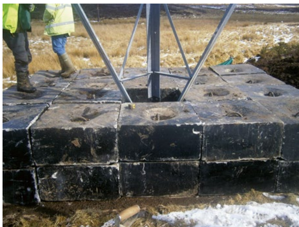
Figure 13.63 Foundation upgrade – Use of precast concrete blocks.
