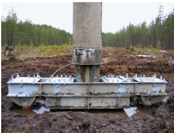
Figure 13.66 Foundation upgrading using steel screw piles and steel beam.
