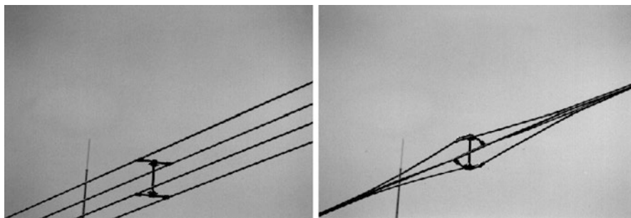
Figure 10.77 Example of quad bundle before and during short-circuit test at 50 kA, showing distortion of the subconductors. One flexible spacer at mid-span (Courtesy Pfisterer/Sefag).
