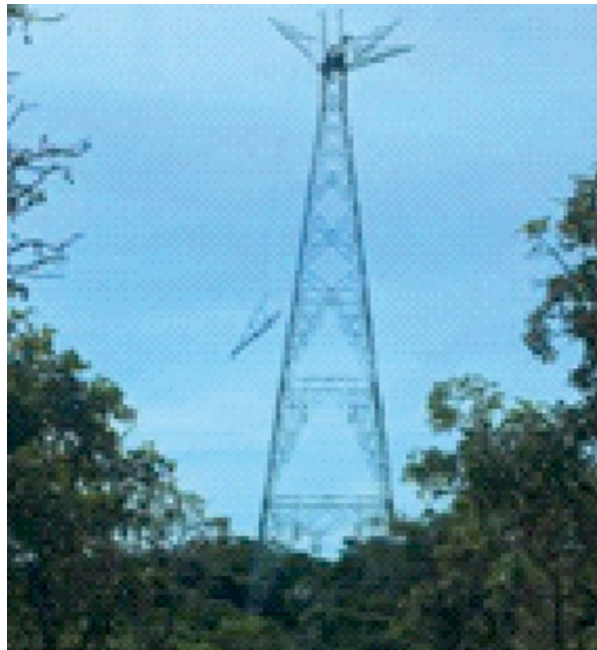
Figure 15.17 Section Method – a cross arm section of a self-supporting suspension tower is erected using a gin pole.
