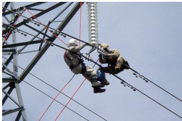
Figure 10.51 Installation of a vibration recorder on a live line.
