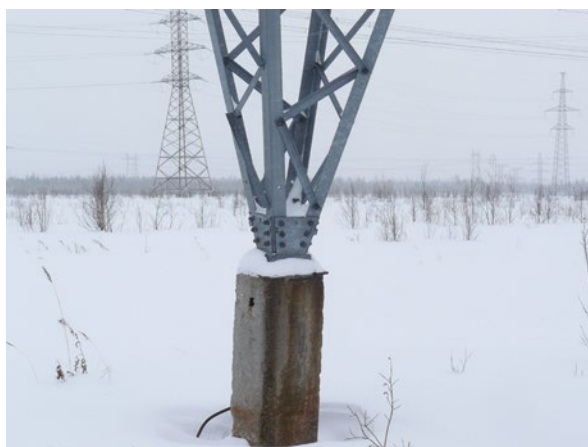
Figure 13.23 Pre-cast concrete pile – Portal guyed tower mast base.
