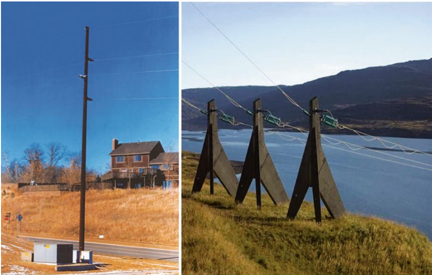
Figure 12.9 Wood OHL Supports.
