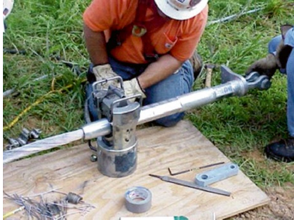
Figure 9.30 Compression of a dead end clamp.
