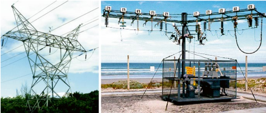
Figure 11.15 Test tower ( left ) and example of a mobile test station ( right ) installed close to the sea for acceleration purposes (Cigré WG B2.03 2007).
