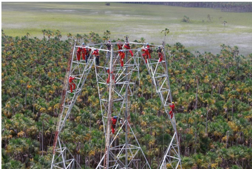
Figure 12.11 Workers on the support during tower erection.
