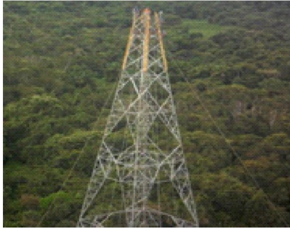
Figure 15.15 Build-up Method/Complementary -Manual erection of the upper part of a self-supporting tower aided by gin poles; tower height exceeded crane capacity range.
