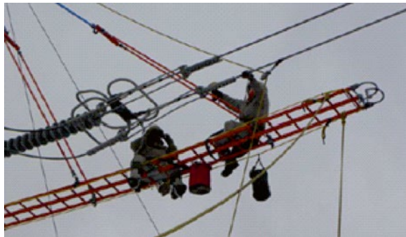
Figure 9.161 Installation of bolted shunts on an energized line using barehanded methods.
