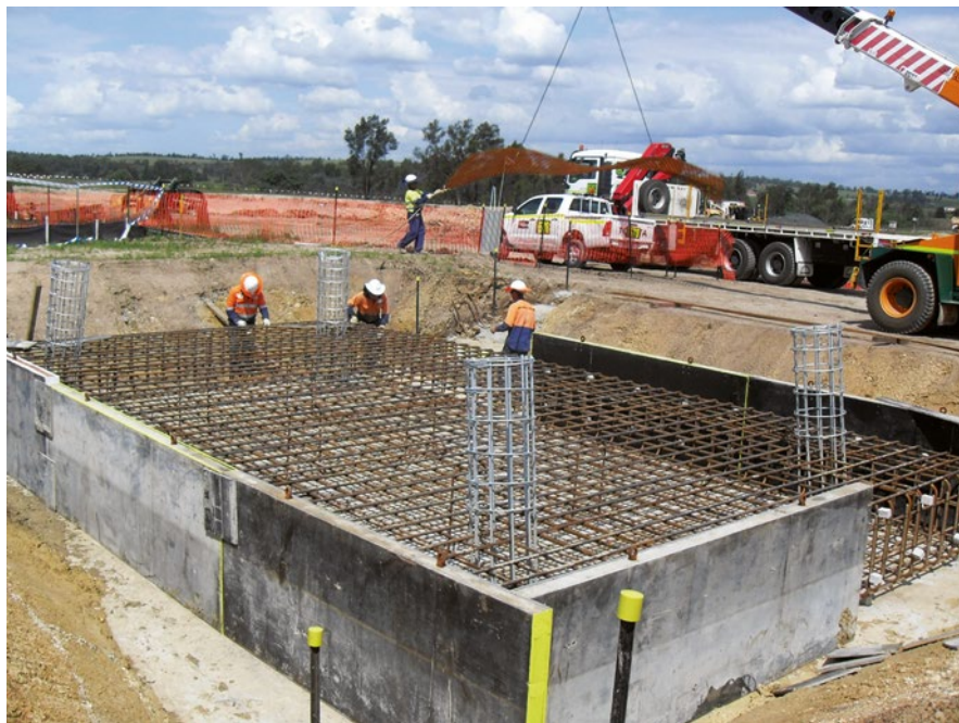
Figure 13.1 Installation of a 330 kV reinforced concrete raft foundation.
