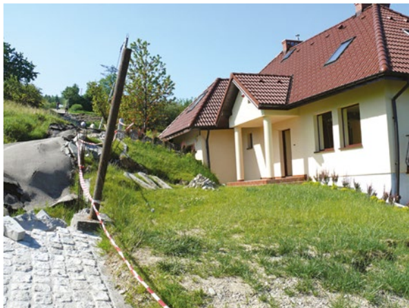
Figure 15.12 Landslide causing destruction of a road, a house and a tower on a 110 kV OHL.
