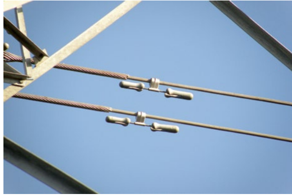
Figure 10.37 Stockbridge type vibration dampers.
