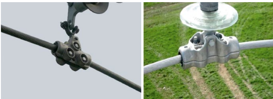
Figure 9.50 Two different ES type suspension clamps.
