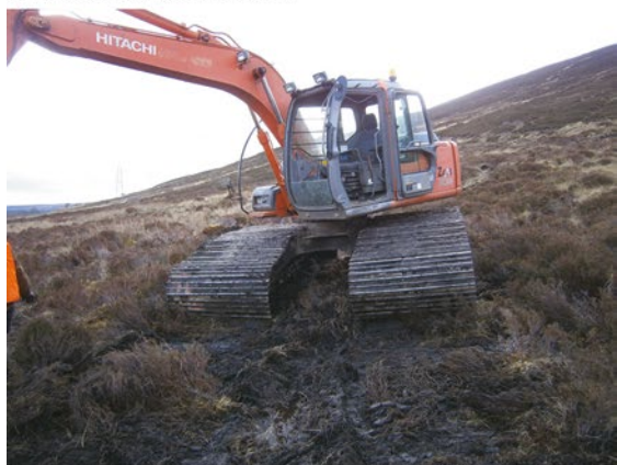
c) Use of low ground pressure excavator to reduce impact on peat soils
