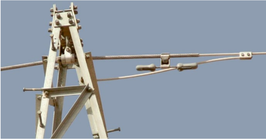
Figure 9.34 Vibration damper of a shield wire installed inside the earthing loop.
