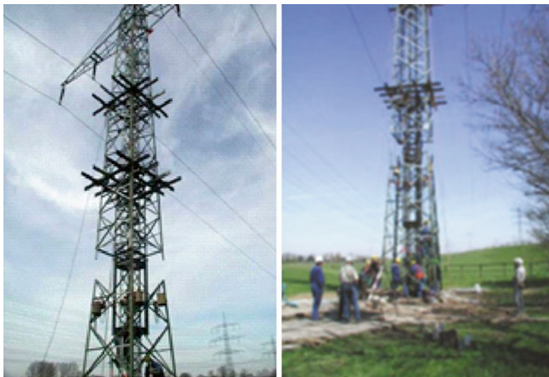
Figure 18.9 Increasing Structure Height.
