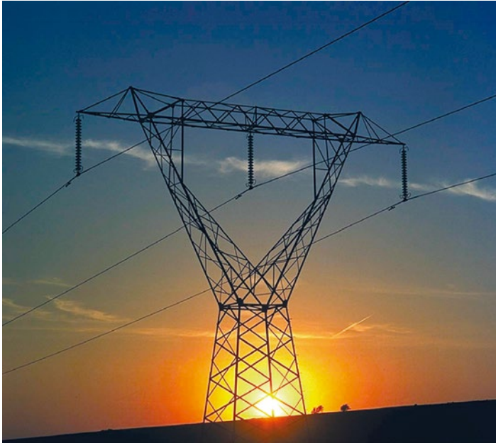
Figure 17.2 220 kV single circuit lattice steel tower.
