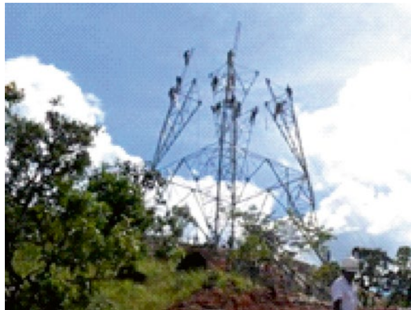
Figure 15.14 Build-up Method - Manual erection of a self-supporting tower aided by gin poles, in a mountainous area; no access for cranes; no place for preassembling.
