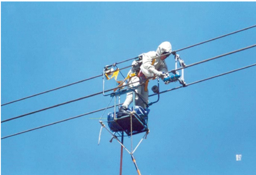
Figure 9.31 Hot line installation of a vibration recorder.
