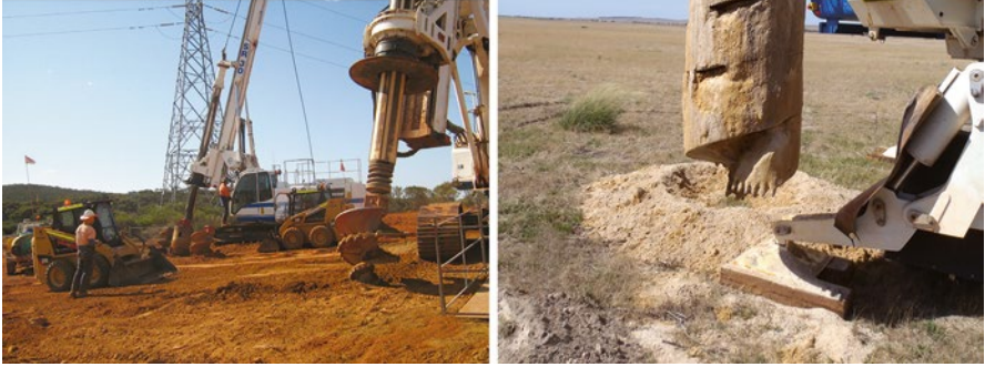
Figure 13.49 Installation of Bored piles.
