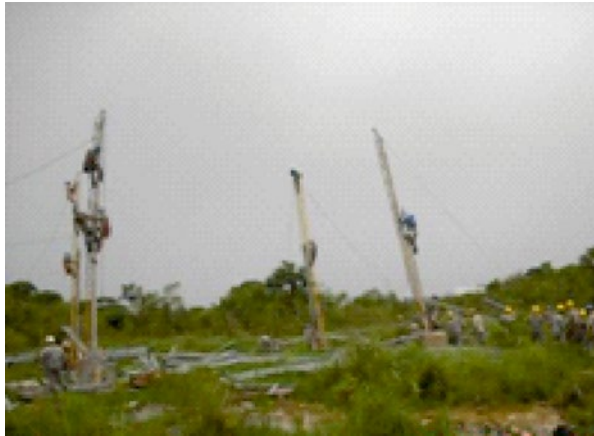
Figure 15.13 Build-up Method - Manual erection of a self-supporting tower aided by gin poles, in a swampy area; no access for cranes; no place for preassembling.
