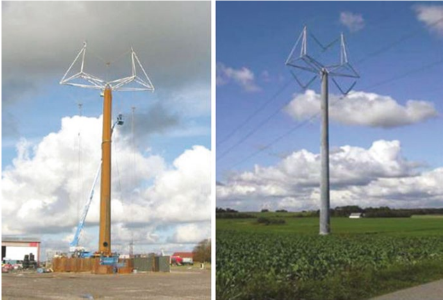
Figure 12.83 400kV TL Aarhus/Aalborg - Denmark.
