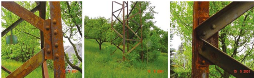
Figure 12.104 Corroded members.
