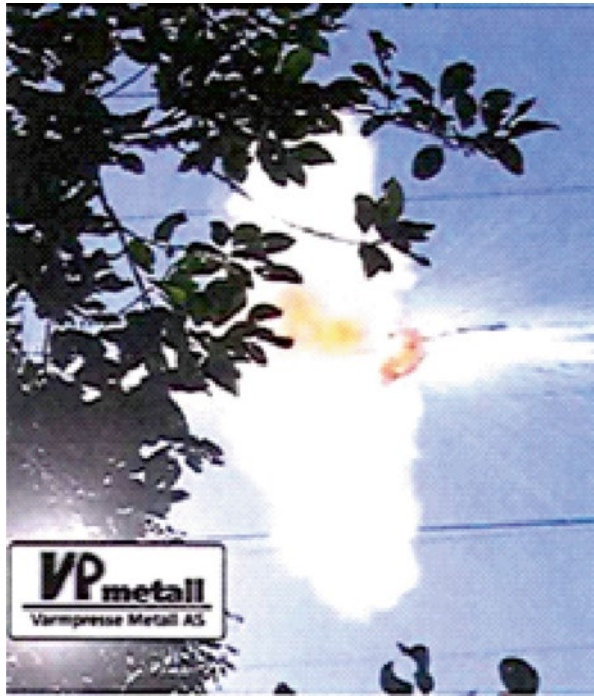
Figure 9.151 Detonation of an implosive joint during installation.
