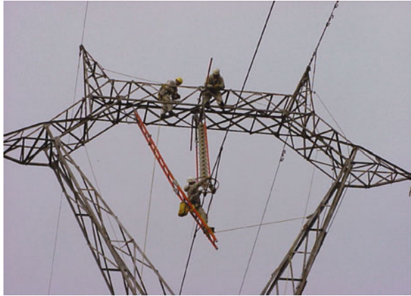
Figure 16.11 Changing 220 kV I-string insulator using bare hand techniques (Spain).
