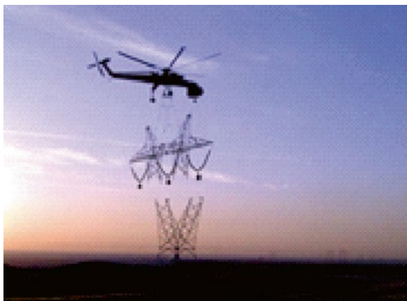
Figure 15.23 Section Method using an Air-Crane – mid sections of a tower are preassembled on the ground and then lifted, flied off and mounted by the S-64 Erickson air-crane; linemen not necessarily required to assist up to this point.
