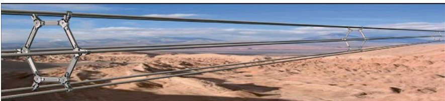
Figure 10.56 Spacer damper distribution on a hexagonal bundle.
