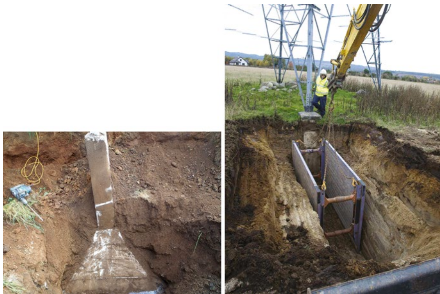
Figure 13.62 Intrusive foundation inspection.
