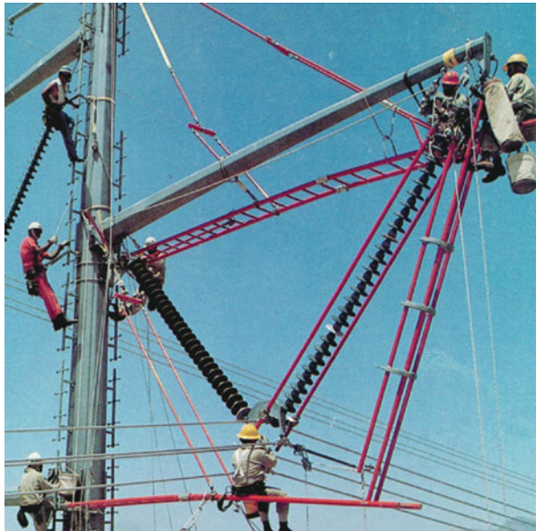
Figure 16.12 Changing a 500 kV V-String Insulator using Bare Hand Techniques (USA).
