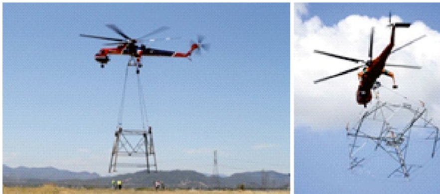
Figure 15.23 Section Method using an Air-Crane – mid sections of a tower are preassembled on the ground and then lifted, flied off and mounted by the S-64 Erickson air-crane; linemen not necessarily required to assist up to this point.
