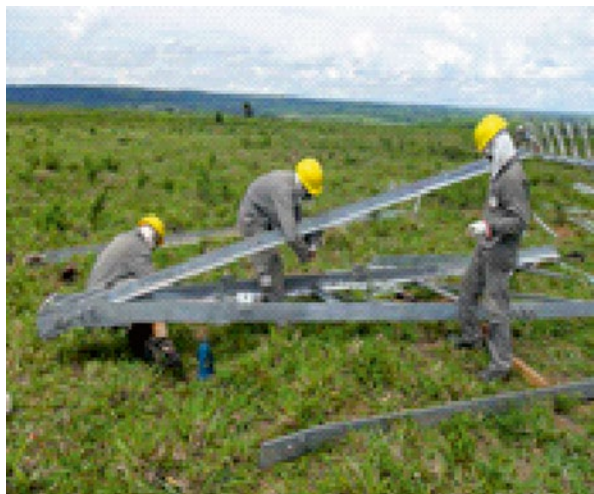
Figure 15.19 Section Method – a cross arm section of a tower is preassembled on the ground; this method speeds up the erection process.
