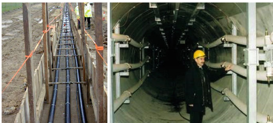
Figure 19.2 Left – one cable system direct buried in soil (from Cigré TB 338, page D.2); Right - two XLPE 400 kV cable systems in a ventilated tunnel, 2×1100 MVA, special application in cities (Berlin, picture APG).
