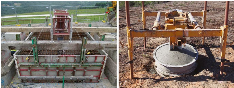
Figure 13.55 Stub setting.
