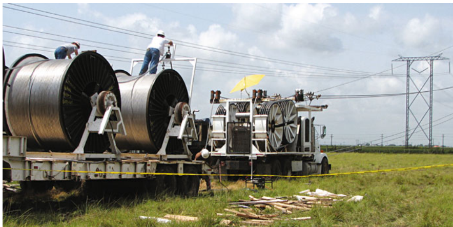
Figure 1.21 Trailer mounted payoffs and a truck mounted bullwheel for tension stringing.
