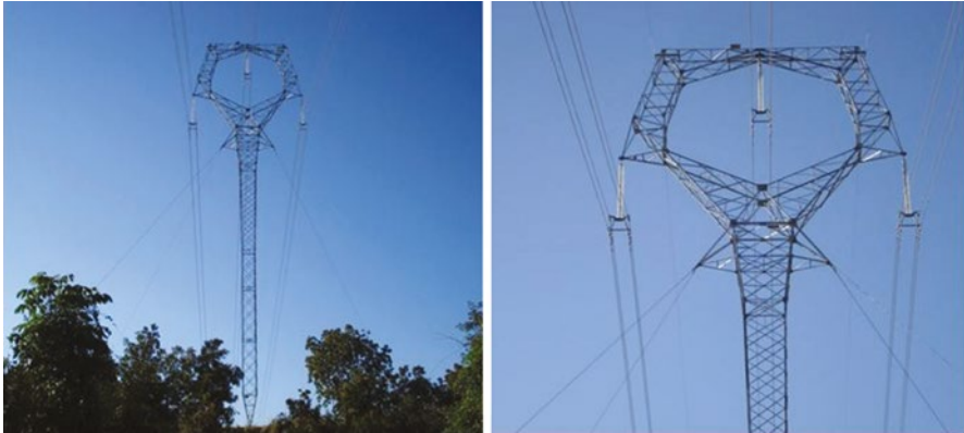
Figure 12.65 500kV Lattice Guyed Monomast Support.
