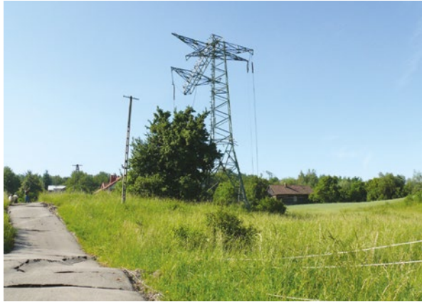
Figure 15.11 Tension tower destroyed and moved down about 14 m on a 110 kV OHL.
