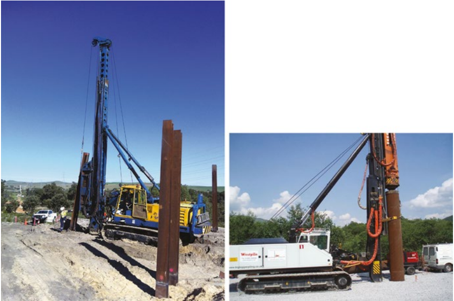
Figure 13.50 Installation of Driven piles 'H' section (left) and tubular steel (right).
