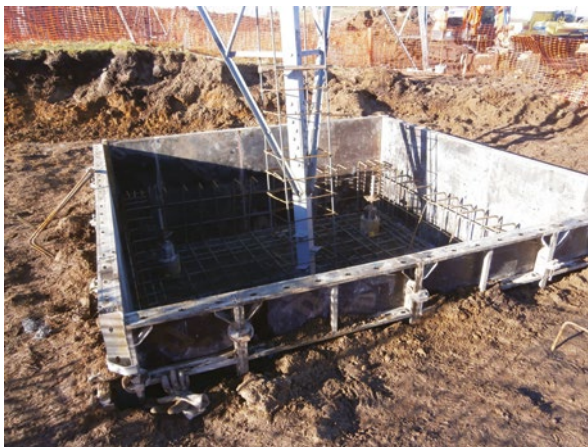
Figure 13.65 Foundation upgrading – Installation of micropile reinforced concrete cap.
