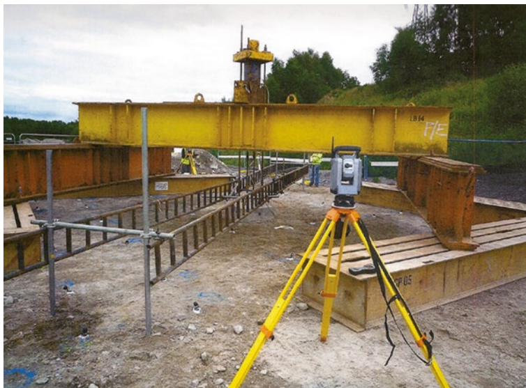
Figure 13.40 Full-scale uplift test arrangement for P&C concrete foundation.
