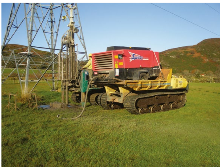
Figure 13.64 Foundation upgrading – Installation of micropiles.
