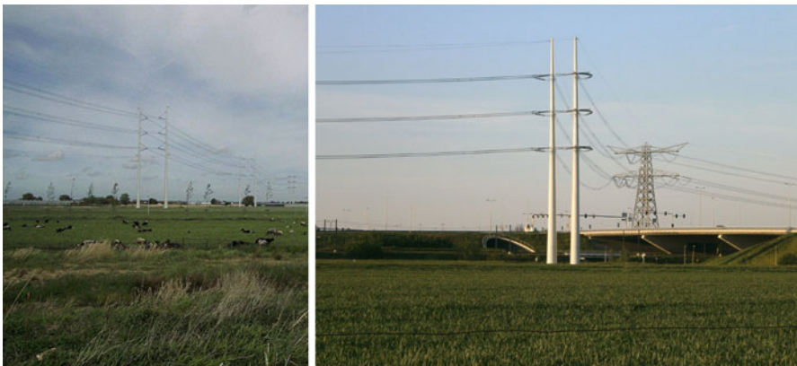
Figure 19.11 Wintrack tower in the Netherlands (APG).
