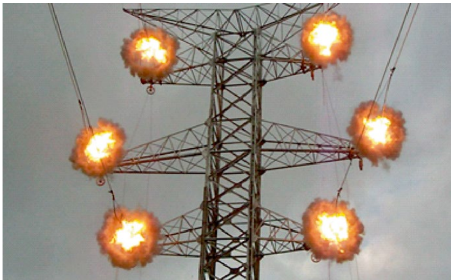
Figure 15.43 Simultaneous installation of multiple implosive type sleeves.
