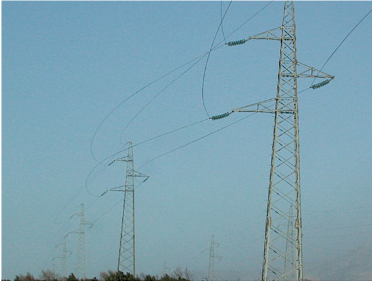
Figure 7.7 Conductors blow out during a Bora event in Croatia, January 2003. From Cigré TB 256 (Photo: F. Jakl).
