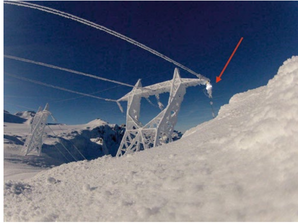
Figure 11.45 Snow flashover across the tension set of a 420 kV line.
