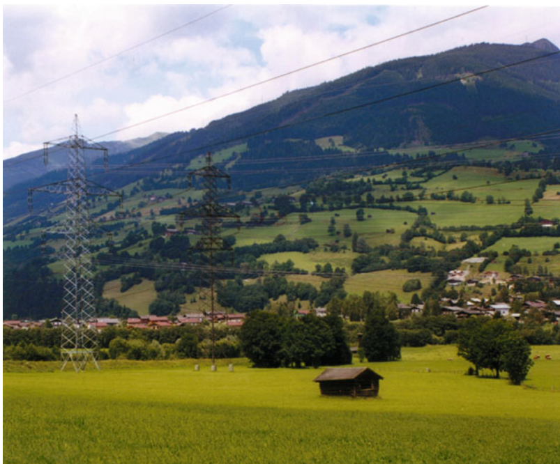
Figure 19.12 Two 400 kV towers can be seen. Left: galvanized steel tower, clearly visible. Right: “camouflage line” with dark green coated tower and conductors, nearly invisible (APG).
