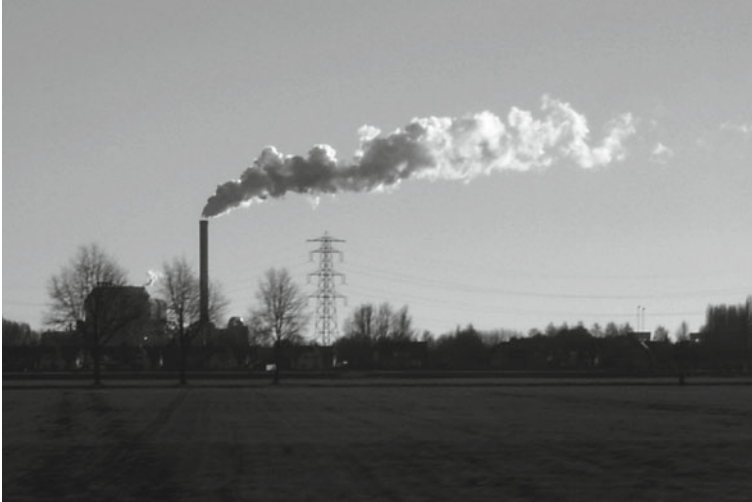
Fig. 2.1 Plume from a smokestack in a stable atmosphere
