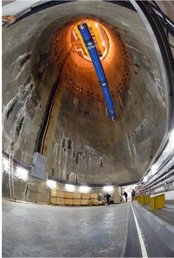
Fig. 3.19 Lowering of cryo-magnet to LHC tunnel via elliptical shaft (CERN photo)
