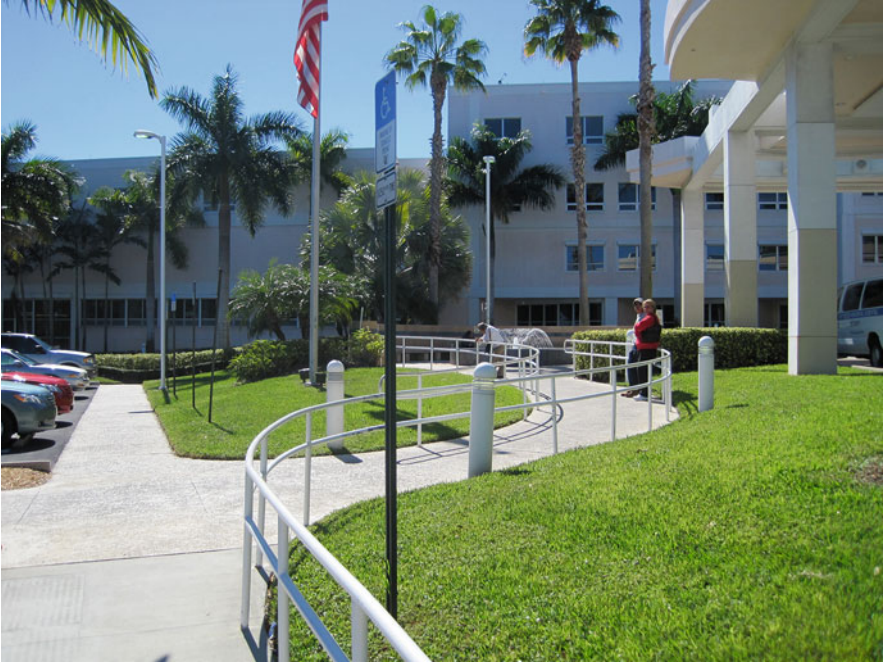
Fig. 5.9 Low physical effort is afforded by making a slightly sloping walkway (as opposed to a steeper ramp) the shortest route from parking to entrance (Photo: Jon A. Sanford)
