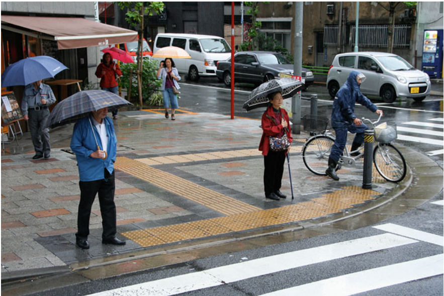
Fig. 5.10 Size and space considerations for wayfinding and mobility include designing spaces so that they are usable by many pedestrians, such as a blended corner (versus two small curb cuts in both directions) that is large enough to accommodate pedestrians with different types of mobility aids (Photo: Jon A. Sanford)
