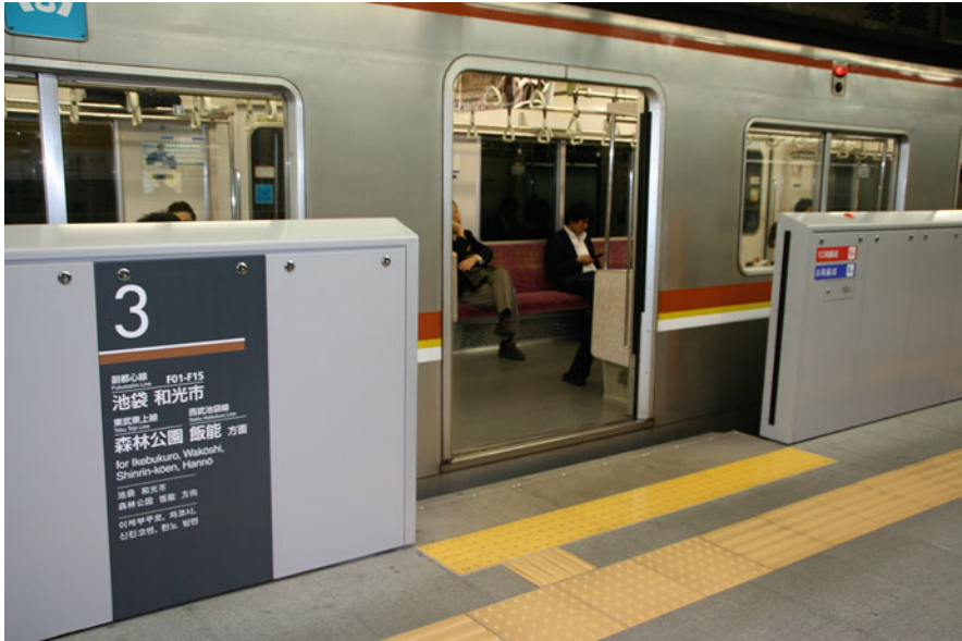
Fig. 5.8 Fail-safe features for wayfinding and mobility can take many forms, including the use of auditory, visual, and tactile information (Photo: Jon A. Sanford)
