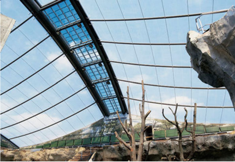
Fig. 3.10 Fully transparent and open in the central part to maximize natural ventilation of the site
