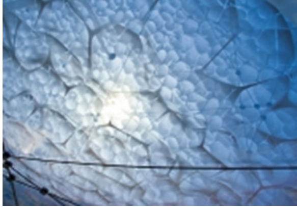
Fig. 3.4 Example of ETFE membrane, the airtight cushion offers shelter while allow light to pass through its transparent form (photo by Niklaus Spoerri)
