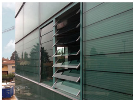
Castel Maggiore tower: building envelope with second active skin and punctual solutions of interactive building envelope
