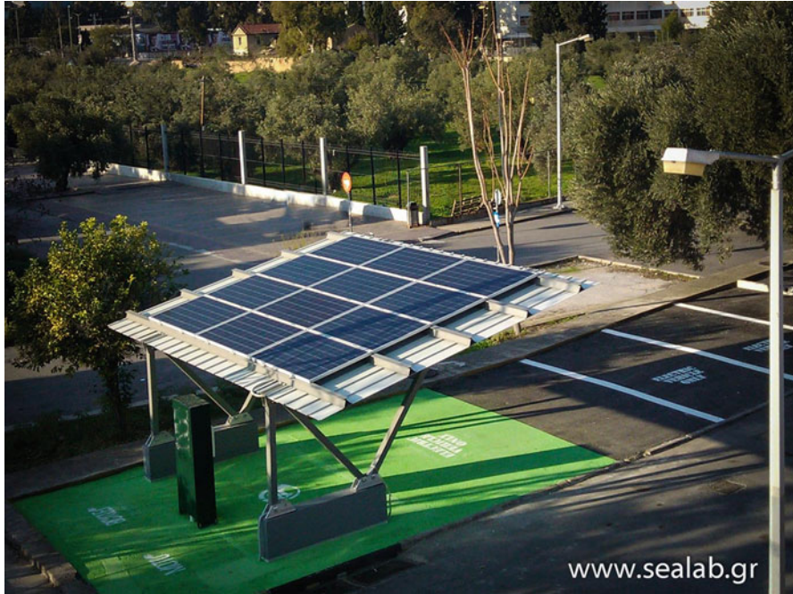
Fig. 37.10 Proposed solar electric vehicle charging station (CARPORT) at SEALAB of Piraeus University of Applied Sciences: general view
