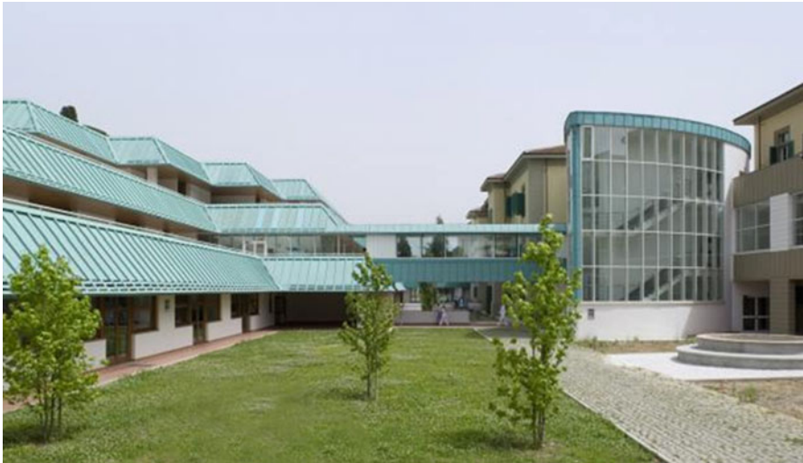
Fig. 1.2 South façade of new part of building
