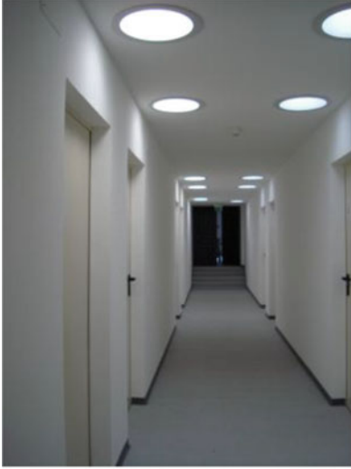
Solar tunnels at the Ion Mincu University of Architecture (left) Photo: personal archive Solar light pipes, at the Berlin Potsdamer Platz Metro Station (right) Photo: Dabbelju CC-BY-SA 2.5
