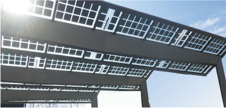
Fig. 3.12 Another solution for PV shelter roof
