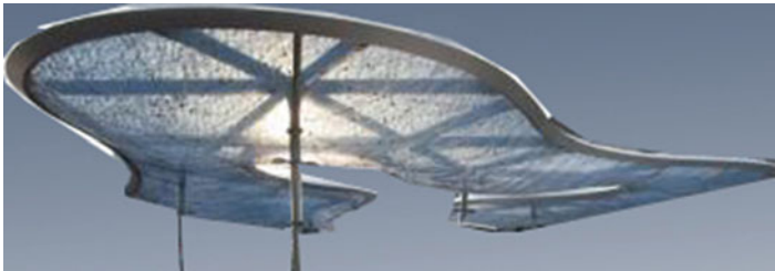
Fig. 3.6 Example of ETFE membrane; the airtight cushion offers shelter while allowing light to pass through its transparent form (photo by Niklaus Spoerri)
