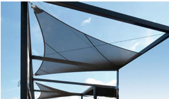
Fig. 3.9 This cover is realized in a stretchable water tight fabric, ensuring easy protection against sun and rain. The stretchable fabric bends and strains under tension. It is ultralight (only 3 kg) and easily washed. The corner fixation hooks are automatically loosened in case of strong gusts or excessive tension
