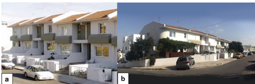
Fig. 21.1 Terrace building under study: (a) south-west view; (b) north-east view
