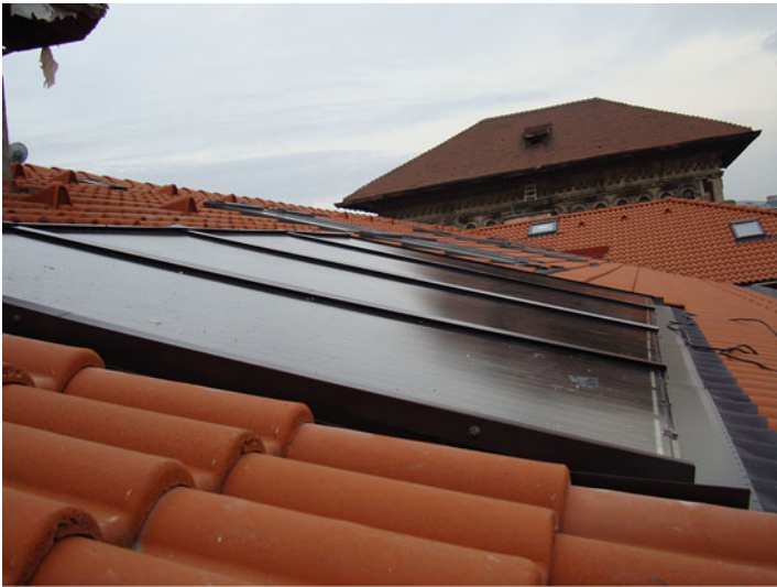
BIPV on the roof of the historic building of the Ion Mincu University of Architecture and Urbanism, Bucharest, Romania Photo courtesy Silviu Gheorghe
