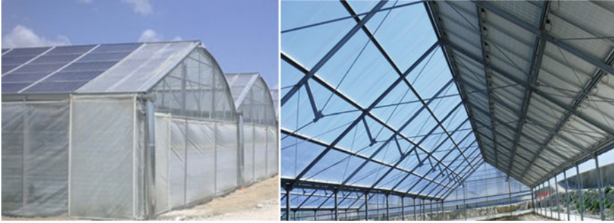
Fig. 16.2 Rounded-roof solar greenhouse ( left ) and slanted-roof solar greenhouse ( right ) [18, 19]
