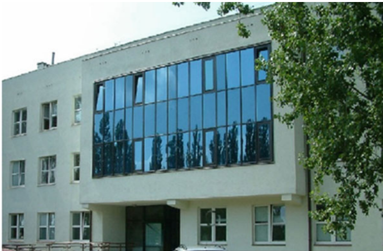
Fig. 1.16 Torun Hospital 100 mm exterior insulation
