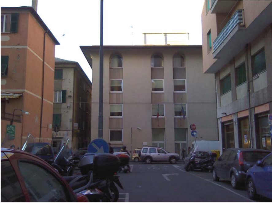
Fig. 45.1 South façade of INPS building in Genoa Sestri Ponente
