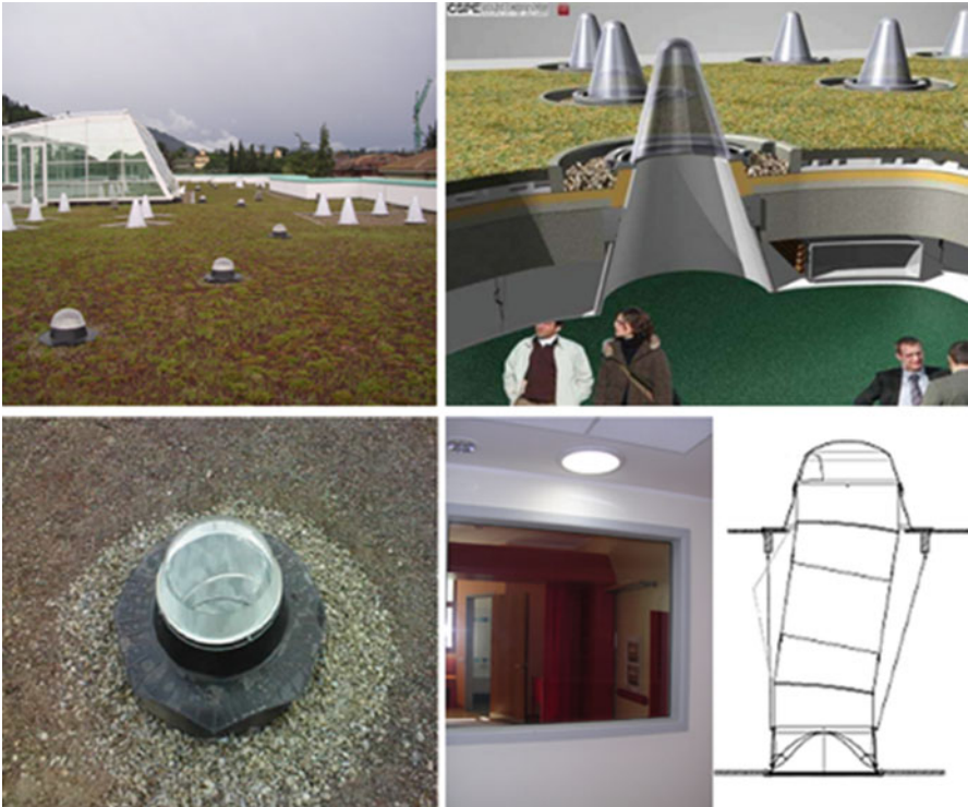
Fig. 1.4 Solar pipes and skylights
