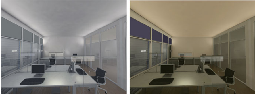
Fig. 58.2 Lighting of an office room. General lighting by transparent LED luminaires integrated into upper area of windows and partitions, light directed toward reflecting ceiling. Task lighting by transparent LED floor lamps. Left : Morning; vertical illuminance 1000 lx, daylight white (6000 K). Right : Evening; vertical illuminance 300 lx, warm white color temperature (3000 K)
