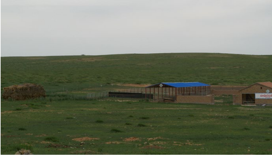
Fig. 4.7 Newly constructed feed stall thanks to the government subsidies in Xinlinhot, Inner Mongolia. (Photo by Li Yang, 2013)
