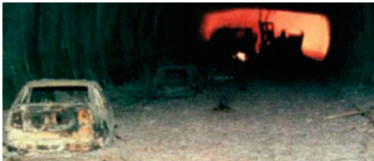
Fig. 1.10 The Tauern Tunnel fire. The main site in the rear burned at over 1000°C. A thick coat of foam covers the ground and parts of the roof hanging down against the fiery background (source http://www.landroverclub.net )
