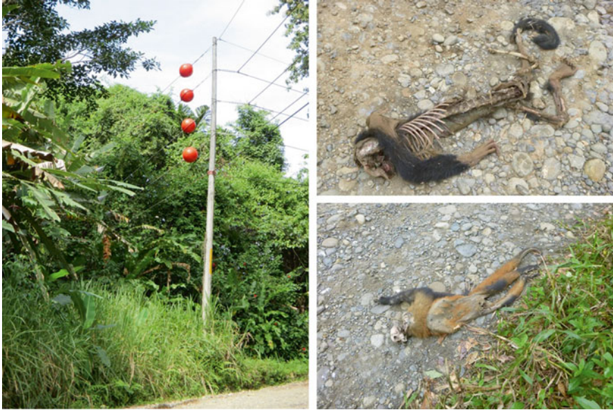
Fig. 3 Inferred electrocution events involving Alouatta palliata (top right) and Ateles geoffroyi (bottom right). Subsequently, wildlife barriers (orange spheres, left photo) were installed at this site. Photos by P. Vangoidsenhoven (right) and the author (left)
