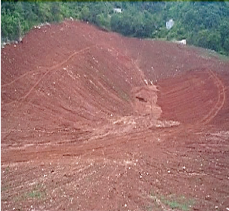
Fig. 3 Untreated top-soil added to this open-cast bauxite mine had been stored (unmaintained) prior to spreading to increase infiltration and facilitate revegetation. Here the process is compromised by wind and water erosion after spreading, and hence is unsuccessful. Adapted from: Google Maps
