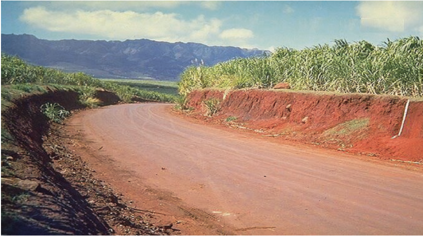
Fig. 15 Top-soil should be stored low (<2 m in height) and planted with fibrous rooted (grassed) vegetation as above
