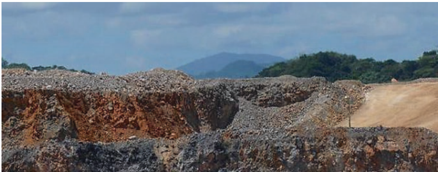
Fig. 4 Pueblo Viejo Mines, Dominican Republic showing weak soil structure caused by low levels of organic matter. Acidic conditions prevent the buildup of organic matter. Reddish oxidized zone in sulfidic waste rock occurred after atmospheric exposure and contact with moisture. Anderson and Cobb (2008) noted that as the surface water reacts with the exposed pyrite, the pH of the surface water decreases and further reacts with pyrite, causing the pyrite to oxidize rapidly. Lower pH can increase the speed of oxidation (Anderson and Cobb 2008). Source Barrick Gold
