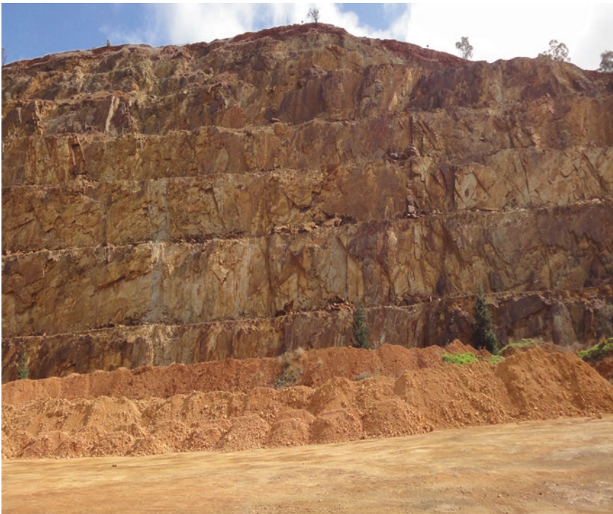
Fig. 1 A decommissioned pyrites mine. Note the contaminated gypsum in foreground after neutralization treatment of the AMD with hydrated lime
