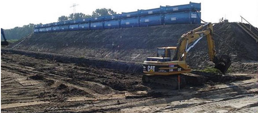
Fig. 2 Dike being monitored with an large scale monitoring system
