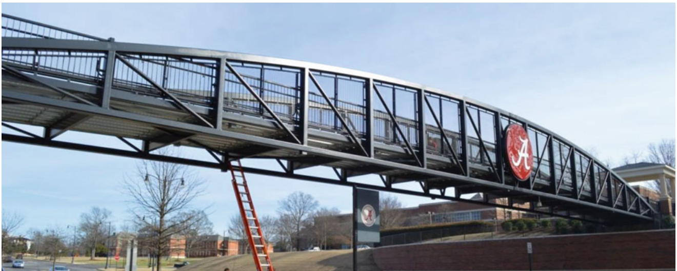
Fig. 28.2 A pedestrian bridge located at the University of Alabama campus
