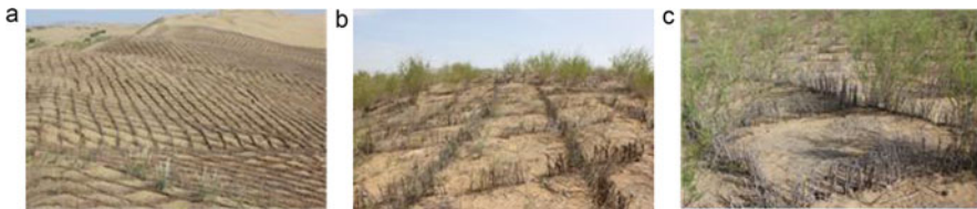
Fig. 24.2 Mobile sand surface stabilized by the checkerboard method, which facilitates development of cyanobacterial biocrusts; conducted in Inner Mongolia, China. Often made of straw, these checkerboards were constructed from twigs of Salix psammophila . (a) Newly made checkerboards on mobile sand dunes. (b) Some of the twigs in the checkerboards developed into new S. psammophila plants which were beneficial to surface stabilization. Cyanobacterial crusts developed in the open spaces within the checkerboards. (c) Dark cyanobacterial crust developing within the checkerboards (Photo by Dunhai Li)
