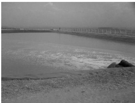
Fig. 4 Depuration lagoon where vinasse is stored at an ethanol and sugar industry (São Paulo, Brazil). Vinasse flow at the moment the pictures was taken was 350 m 3 h -1 . Source The authors
