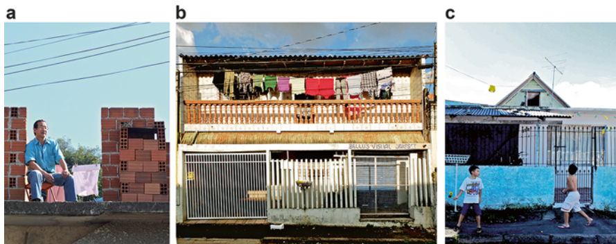
Fig. 5.5 Examples of different housing modifications (Source: Taken by: Federica Natalia Rosati (author))
