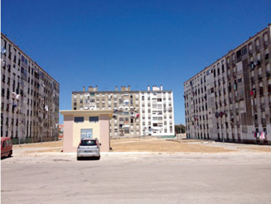
Fig. 2.4 Vale da Amoreira, one of the largest social housing settlements in Portugal, with almost 20,000 ha (Source: Silva 2015)
