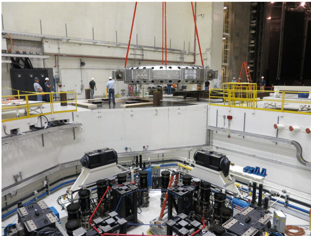
Fig. 16.4 MVF table ( above ) separated from MVF pit ( below ) containing actuators and support structure
