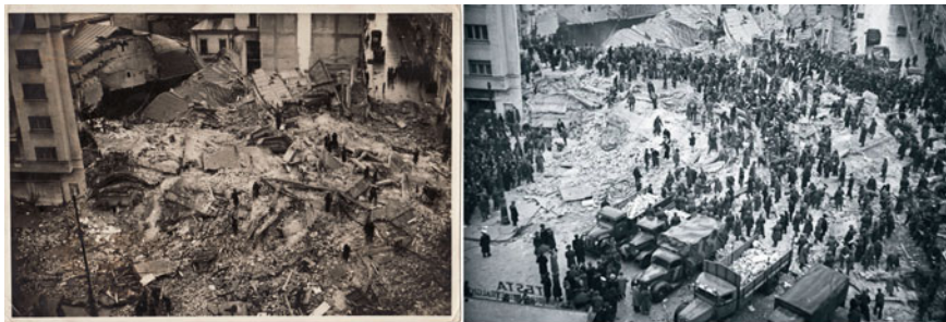
Fig. 3 The collapse of the “Carlton Block” (source http://ro.wikipedia.org )
