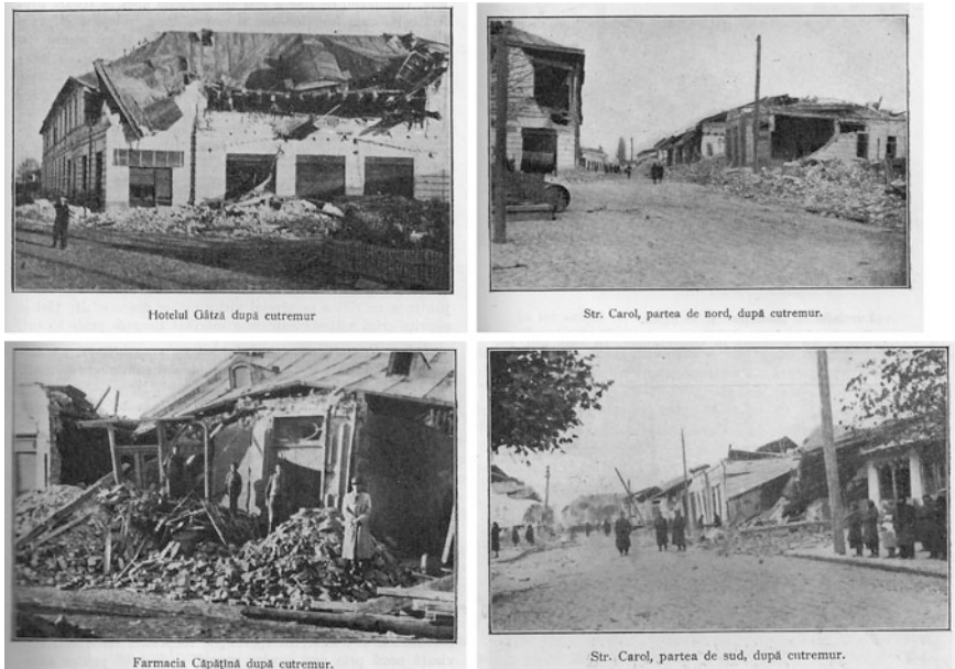
Fig. 6 1940 earthquake damage in Panciu, Romania (Capatana, 1941): Hotel Gatza ( upper left ), Capatana Pharmacy ( upper right ) Carol Street (northern part lower left and southern part lower right )
