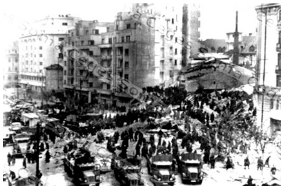
Fig. 13 Carlton building debris in the first period of SAR intervention teams (CEGESOMA Archive)
