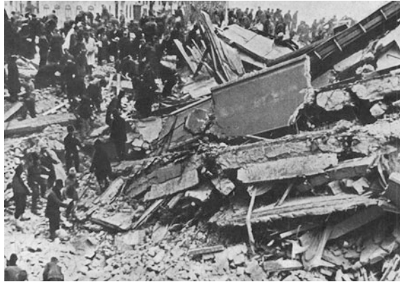
Fig. 10 Carlton building—details of stacked slabs and some parapets or balconies seen from Regala Street (L’Illustration 1940)
