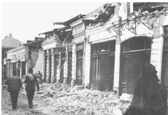
Fig. C.7 Fallen debris on the sidewalk; houses completely damaged (Mândrescu 2008)
