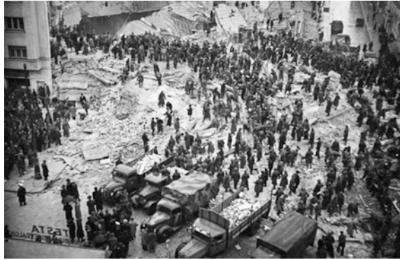
Fig. 14 Carlton building debris in progress of intervention works (Berman 1940)
