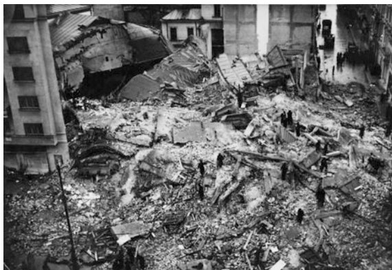
Fig. 9 Carlton building after collapse (Ministry of Propaganda Files 1940)
