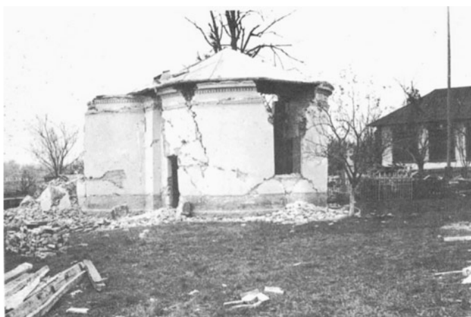
Fig. C.10 A small church in Crucea de Sus completely destroyed (Mândrescu 2008)
