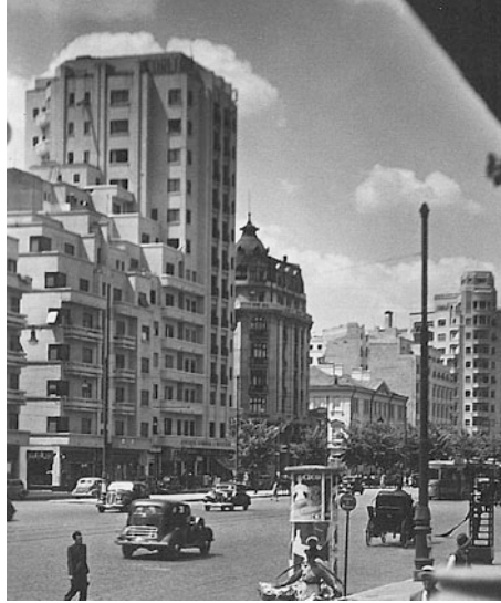
Fig. 1 Carlton building before collapse, seen from S–E (post-card)
