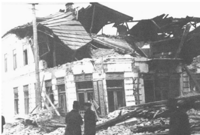
Fig. C.3 Completely destroyed house in Focșani (on I.G. Duca Street) (Mândrescu 2008)
