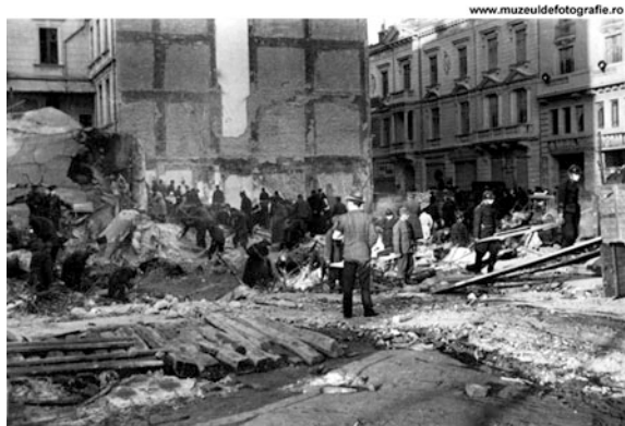
Fig. 17 Carlton building—the site almost cleared of debris (Galmeanu A/Muzeul de fotografie 2015)
