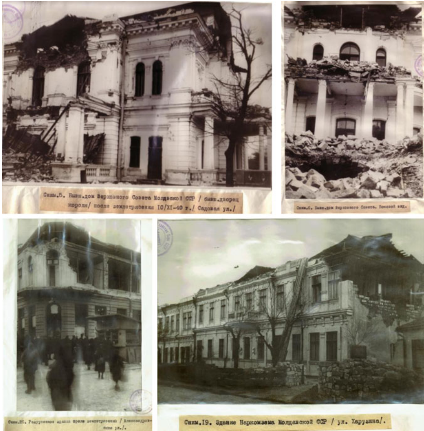
Fig. 7 Buildings in Kishinev severely damaged by the November 10th 1940 earthquake © Institute of Seismology of the Academy of USSR and Institute of Geology and Geophysics Chisinau
