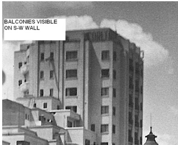
Fig. 6 Detail of S-W balconies that are visible in the Fig. 5 and evaluated by Hangan in 1940 (Hangan 1963; Georgescu 2005, 2007)
