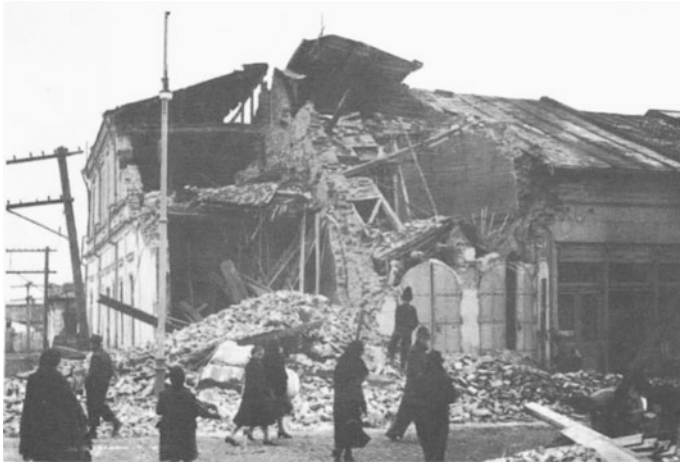
Fig. C.1 Collapsed house in Focșani, looking from east (Mândrescu 2008)
