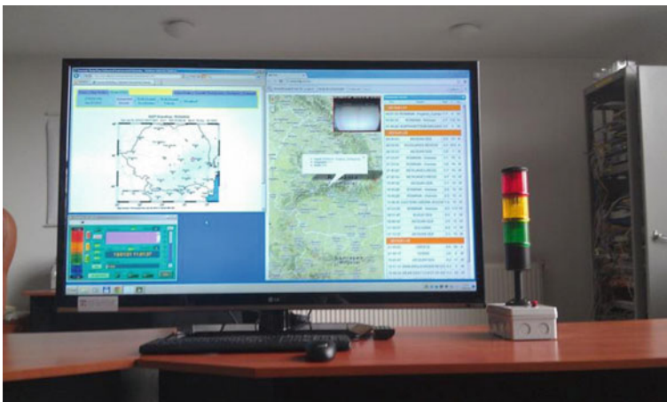
Fig. 10 Earthquake early warning system receiver installed at the emergency response agencies
