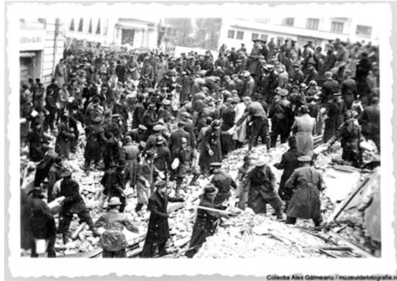
Fig. 15 Carlton building—bare hands army members, civilians and paramilitary removing the debris (Galmeanu A (2015))
