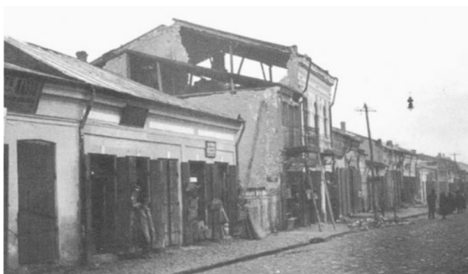
Fig. C.14 View of Adjud Main Street: fallen brick gable of the Blănaru house (Mândrescu 2008)
