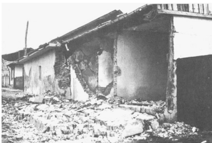
Fig. C.9 Masonry walls fallen towards north (Mândrescu 2008)
