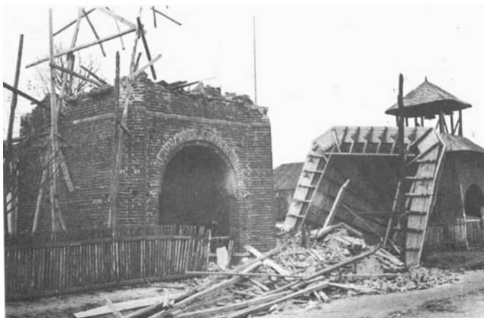
Fig. C.11 The Crucea de Sus steeple roof fallen towards north (Mândrescu 2008)
