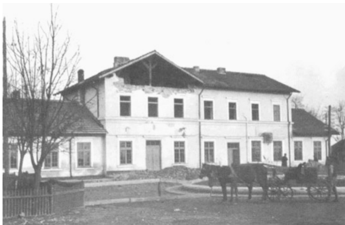
Fig. C.15 City front side of the Adjud railway station—fallen brick gable (Mândrescu 2008)
