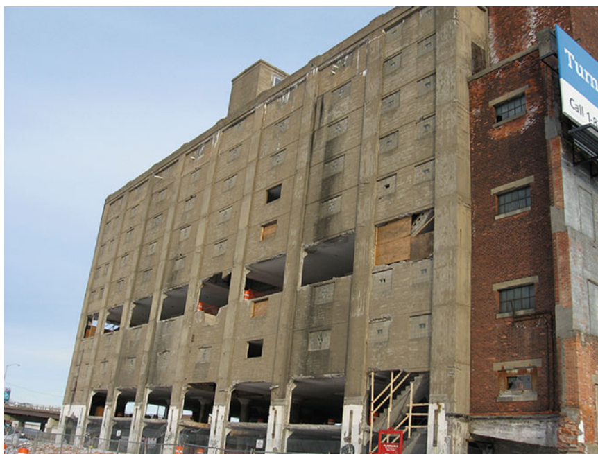
Fig. 28.1 Building view from south west corner
