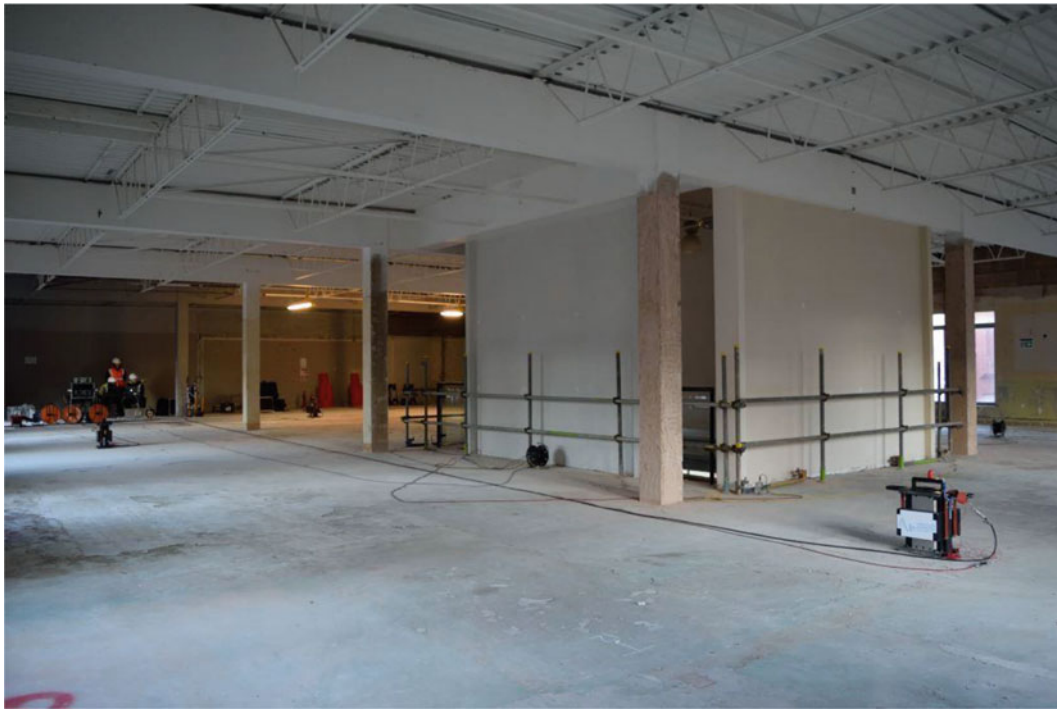
Fig. 34.1 View of the floor
