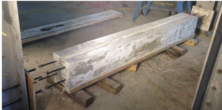
Fig. 33.2 Prestress beam after all strands were released
