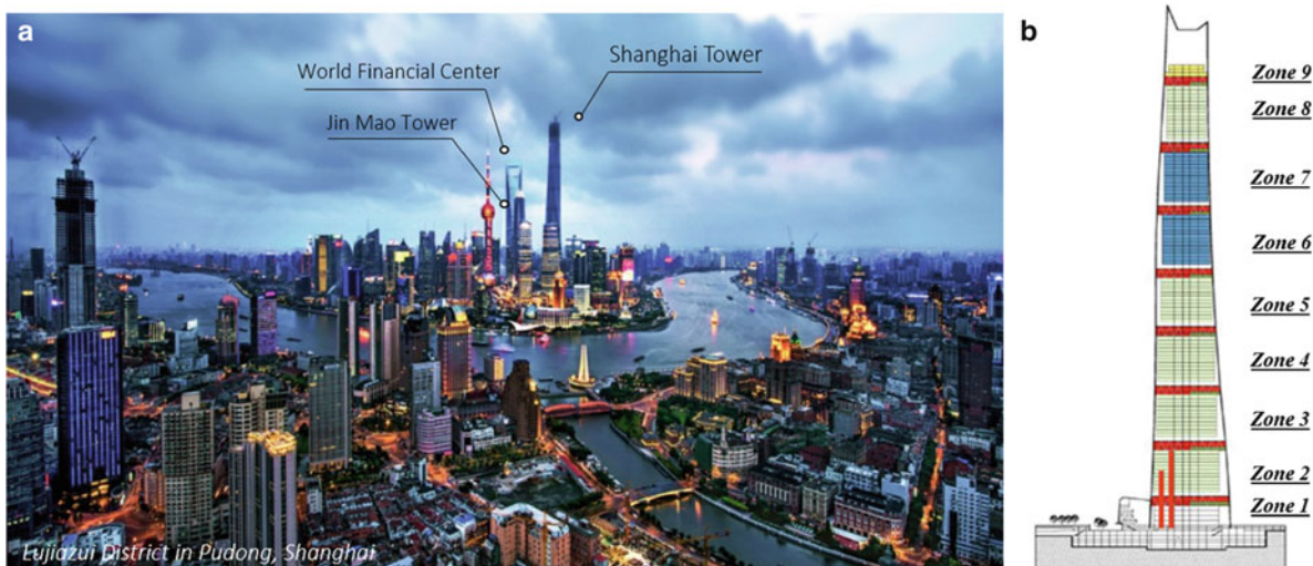
Fig. 16.1 (a) Location of the Shanghai Tower (b) strengthening floors
