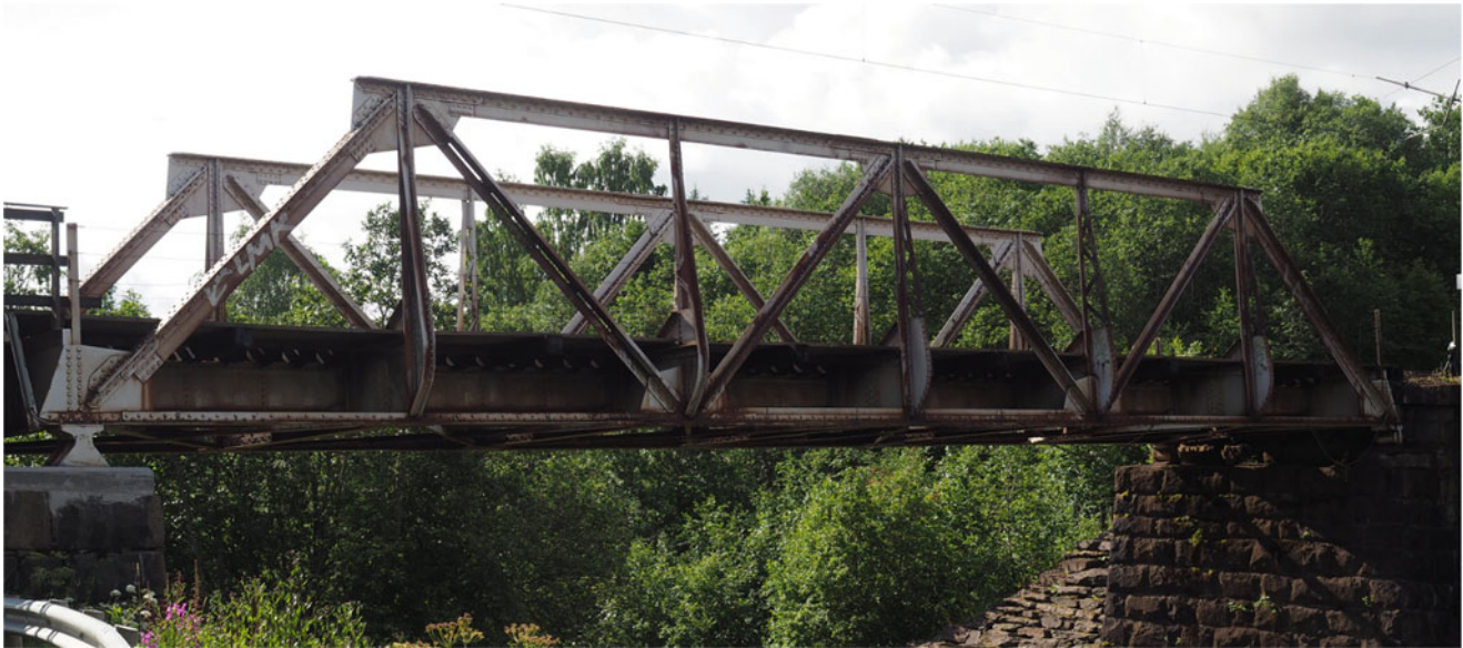
Fig. 23.1 Overview of Lerelva railway bridge
