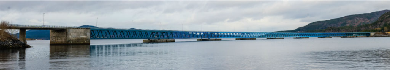
Fig. 22.1 Panorama view of the Bergsoysund bridge
