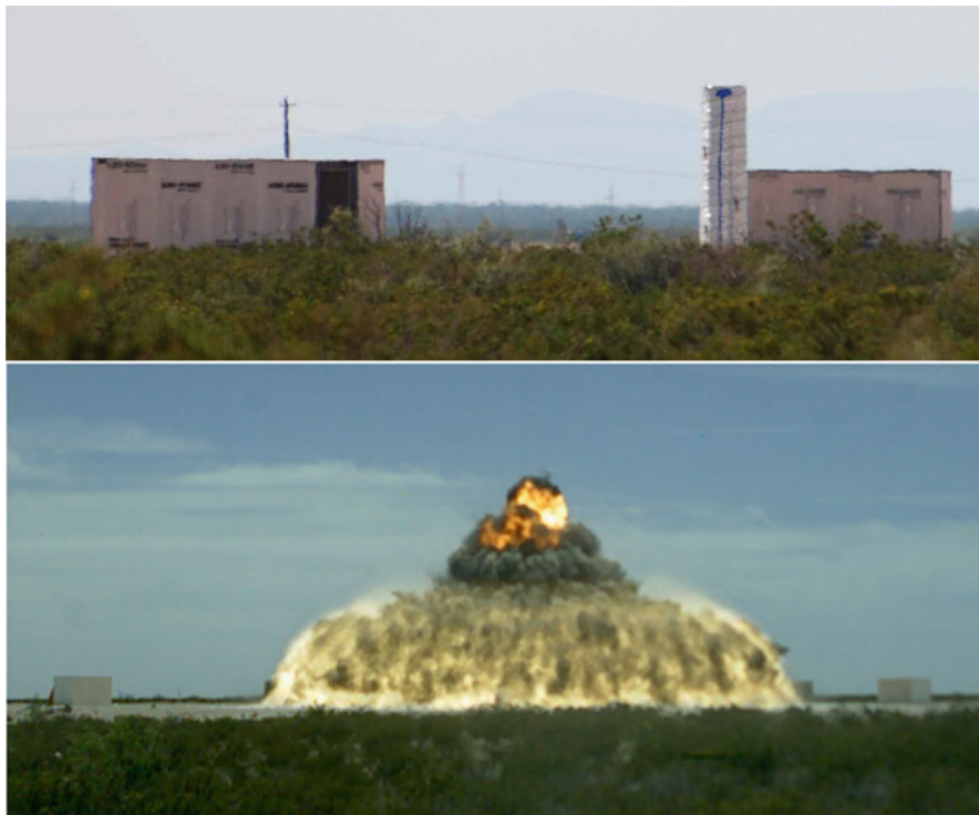
Fig. 13.13 Field testing of stud wall system in blast-resistant module application in arena configuration with charge size of 4,000 kg (9,000 lbs) of ANFO
