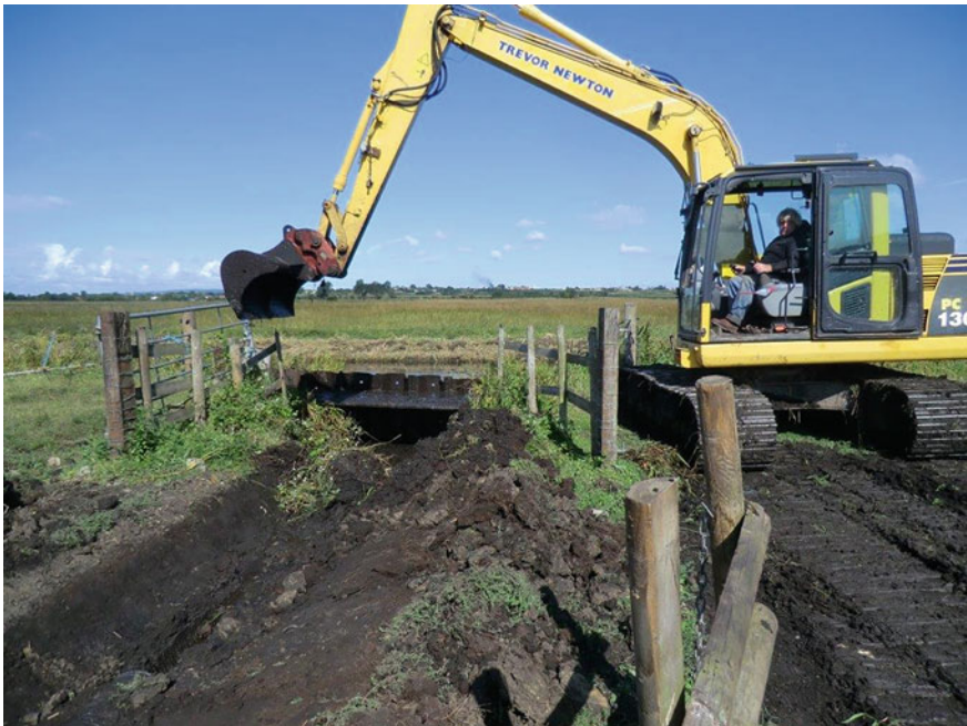
Fig. 5.3 RSPB site preparation for new sluice installation, West Sedgemoor, Somerset UK
