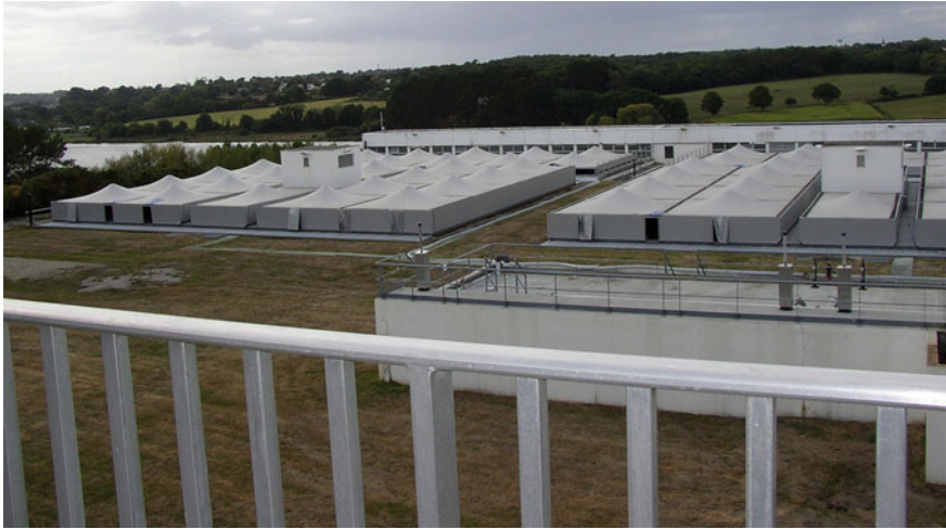
Fig. 11.1 The Drézet drinking water plant, in the Vilaine catchment. Photo Carina Furusho, 16/09/2013
