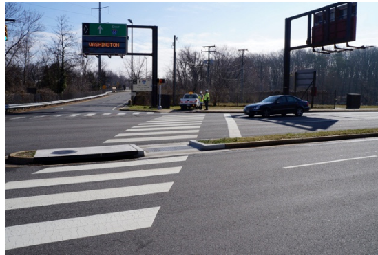
Fig. 1 Wheelchair accommodation in median seen during participant observation that makes street crossing difficult for blind navigators. An architectural change to remove/change this would more easily alleviate this tripping hazard than a technology built to detect and announce it.
