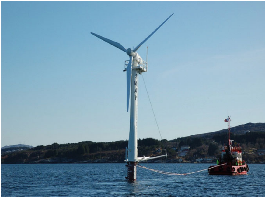
Fig. 47 Sway scaled prototype installed at Kollsnes, Norway
