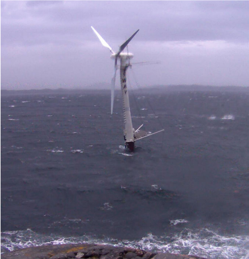
Fig. 48 Installed Sway scaled prototype
