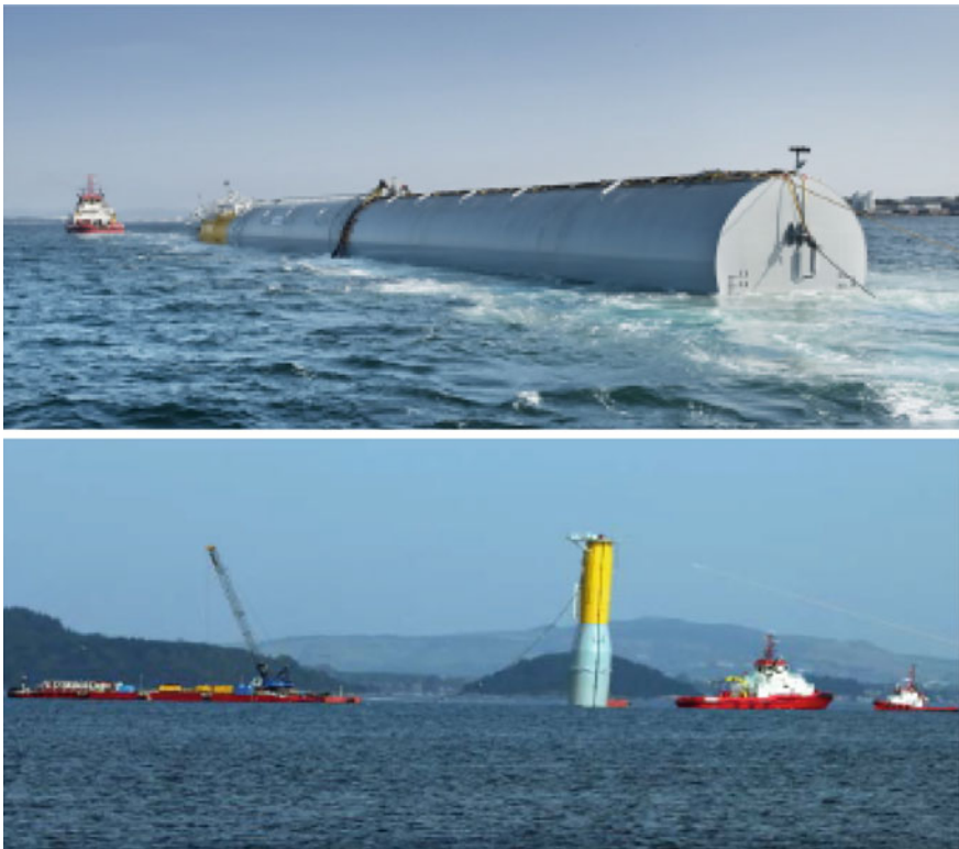
Fig. 19 Towing and upending of Hywind Demo (courtesy of Statoil)
