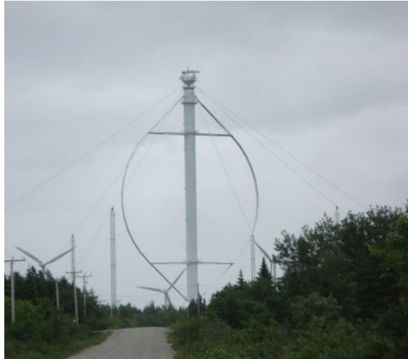
Fig. 8 Éole, the largest VAWT, 110 m height, 60 m diameter, Cap-Chat, Québec. Source Spiritrock4u at en.wikipedia
