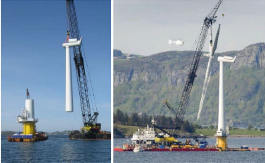
Fig. 20 Assembly of Hywind Demo (courtesy of Statoil)
