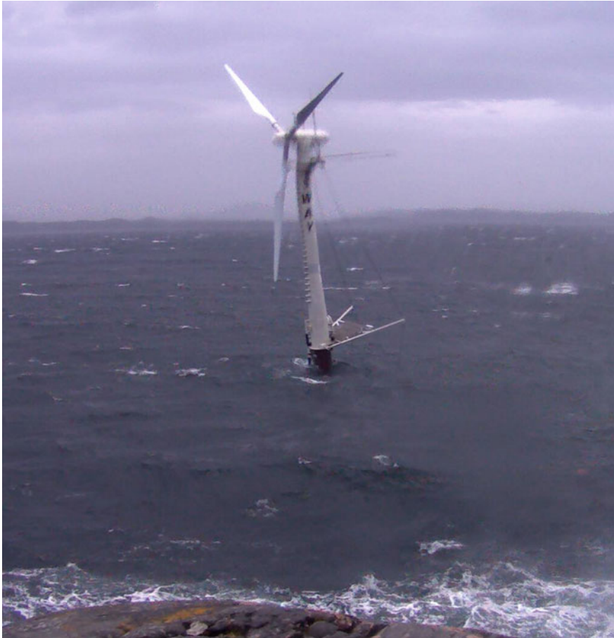
Fig. 48 Installed Sway scaled prototype
