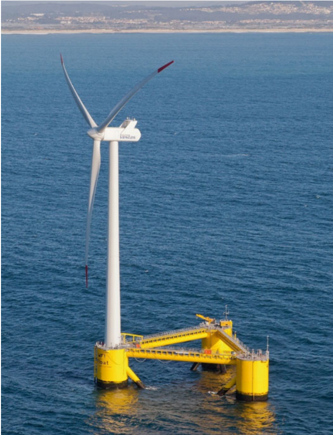
Fig. 2 WF1 prototype operating at rated wind speed in Aguçadoura (Portugal)
