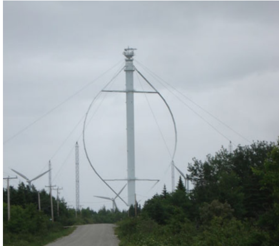
Fig. 8 Éole, the largest VAWT, 110 m height, 60 m diameter, Cap-Chat, Québec. Source Spiritrock4u at en.wikipedia
